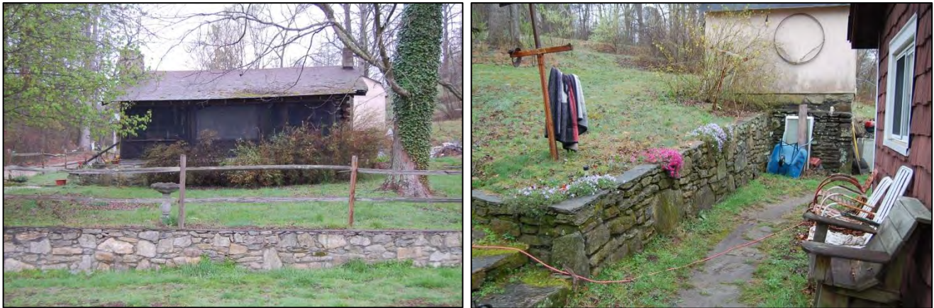
Figure 83. Retaining wall facing Balfour Road, at left; retaining wall behind house, at right
