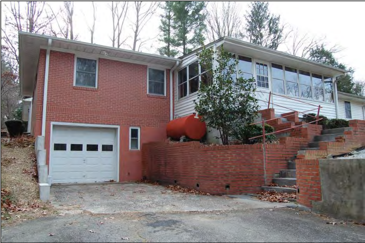
AECOM #96 - 120 May Dr: N front and E side elevations
