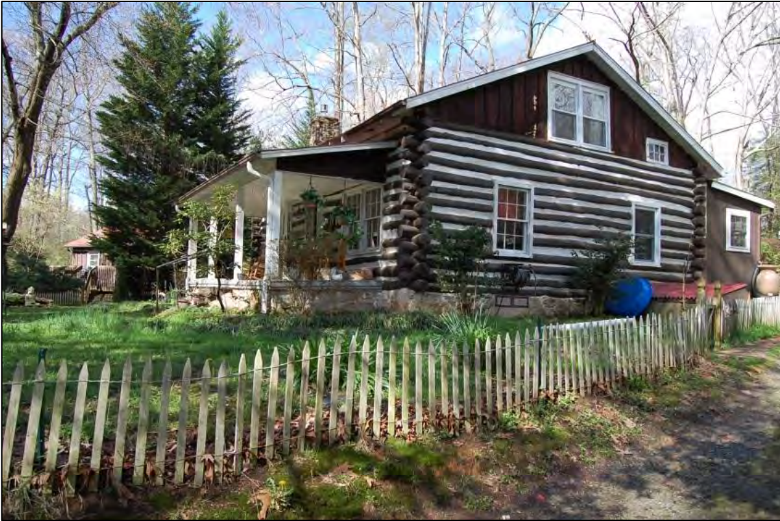
Figure 55. South front and east side elevations of log house; frame cabin visible at far left
