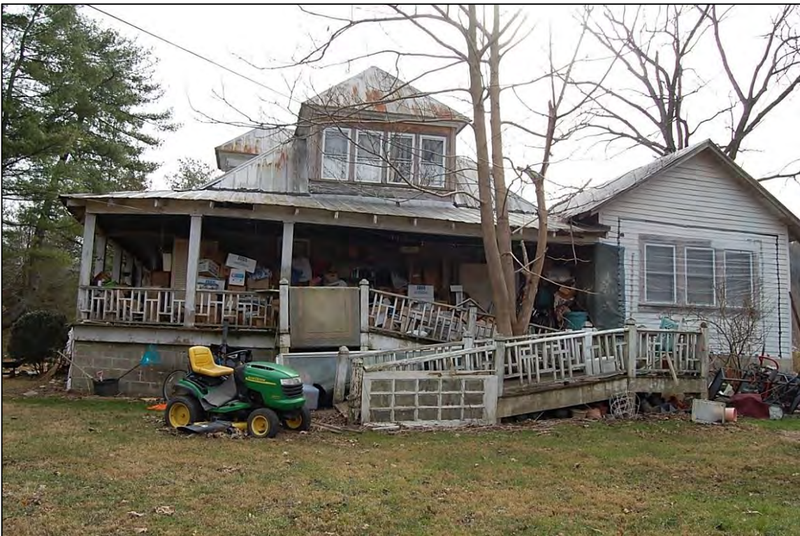
Figure 193. North side elevation with wheelchair ramp in foreground
