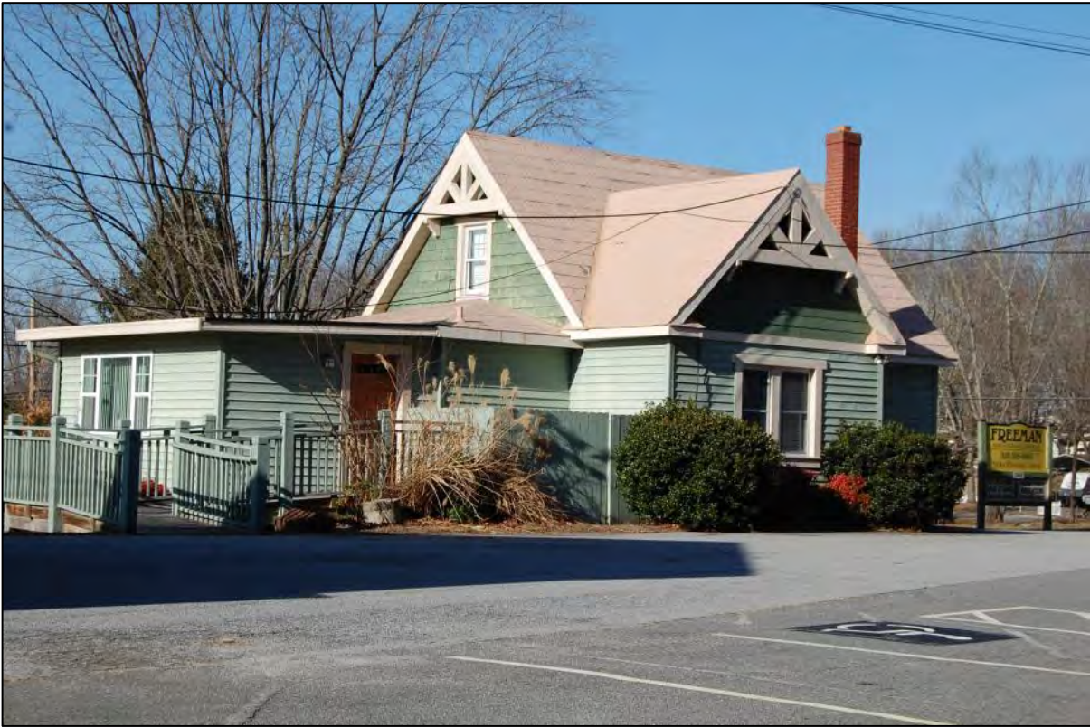
AECOM #15 - 2840 Chimney Rock Rd: E side and S rear elevations of former house
