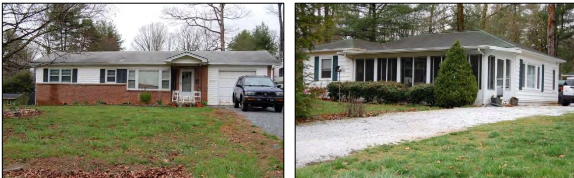
Figure 108. 3118 Florida Drive at left and 3108 Florida Drive at right
