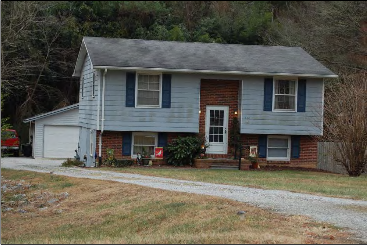
AECOM #62 - 855 Stoney Mountain Rd: N front and E side elevations
