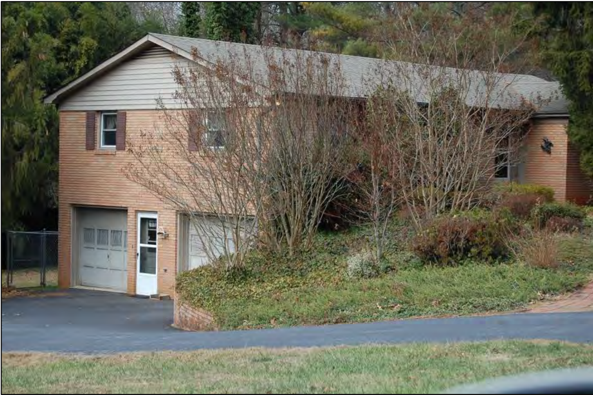
AECOM #100 - 109 Shannon Rd: E front and S side elevations
