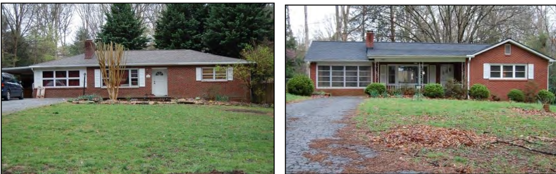
Figure 100. 3209 Cardinal Lane at left and 3159 Cardinal Lane at right
