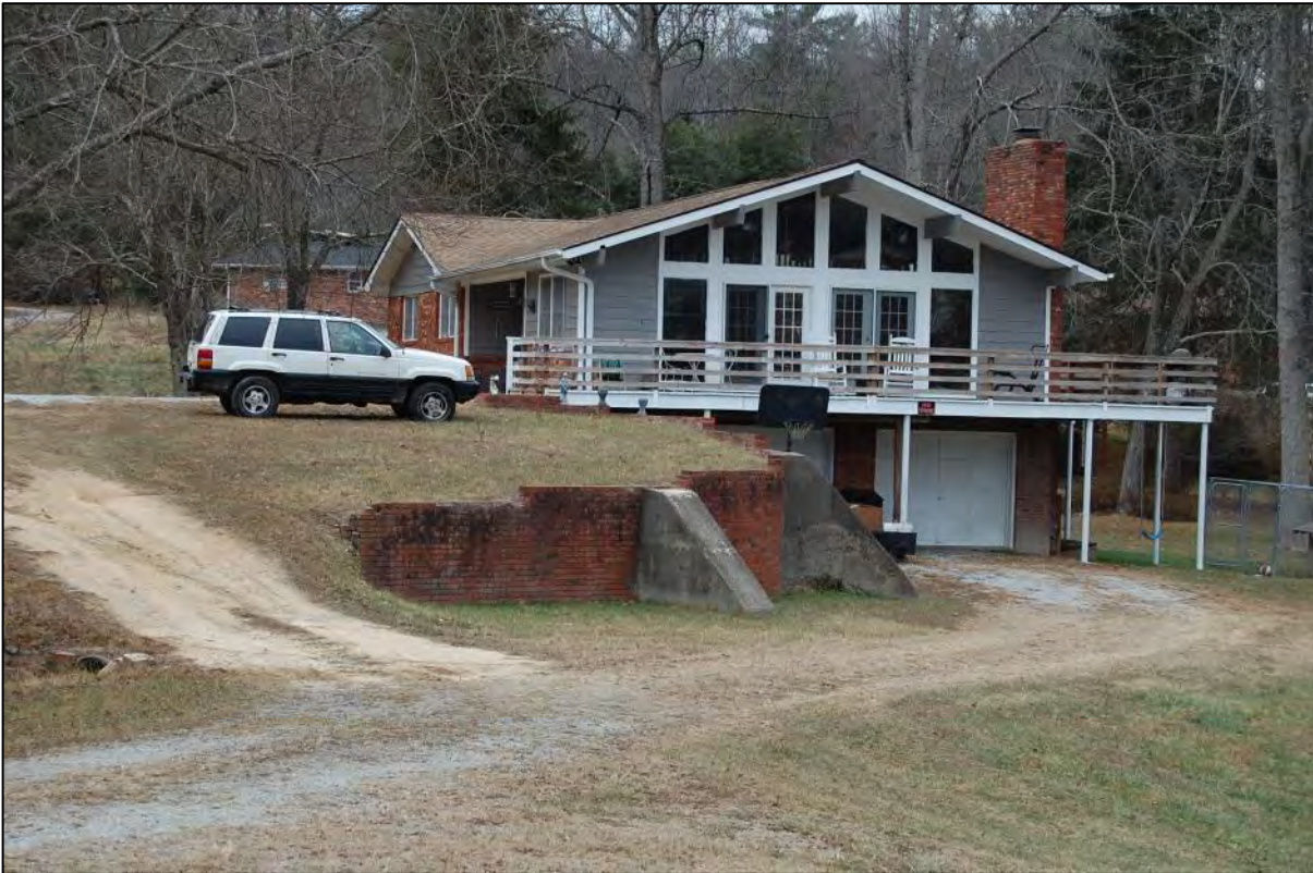
AECOM #64 – 101 Leverette Dr: S front and E side elevations
