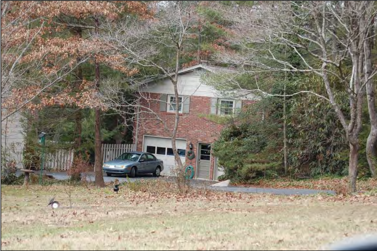
AECOM #121 - 127 Castleton Ln: S side elevation
