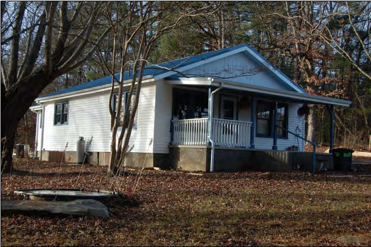
AECOM #49 (HN1935) - 619 Hyder Farm Rd: E front and S side elevations
