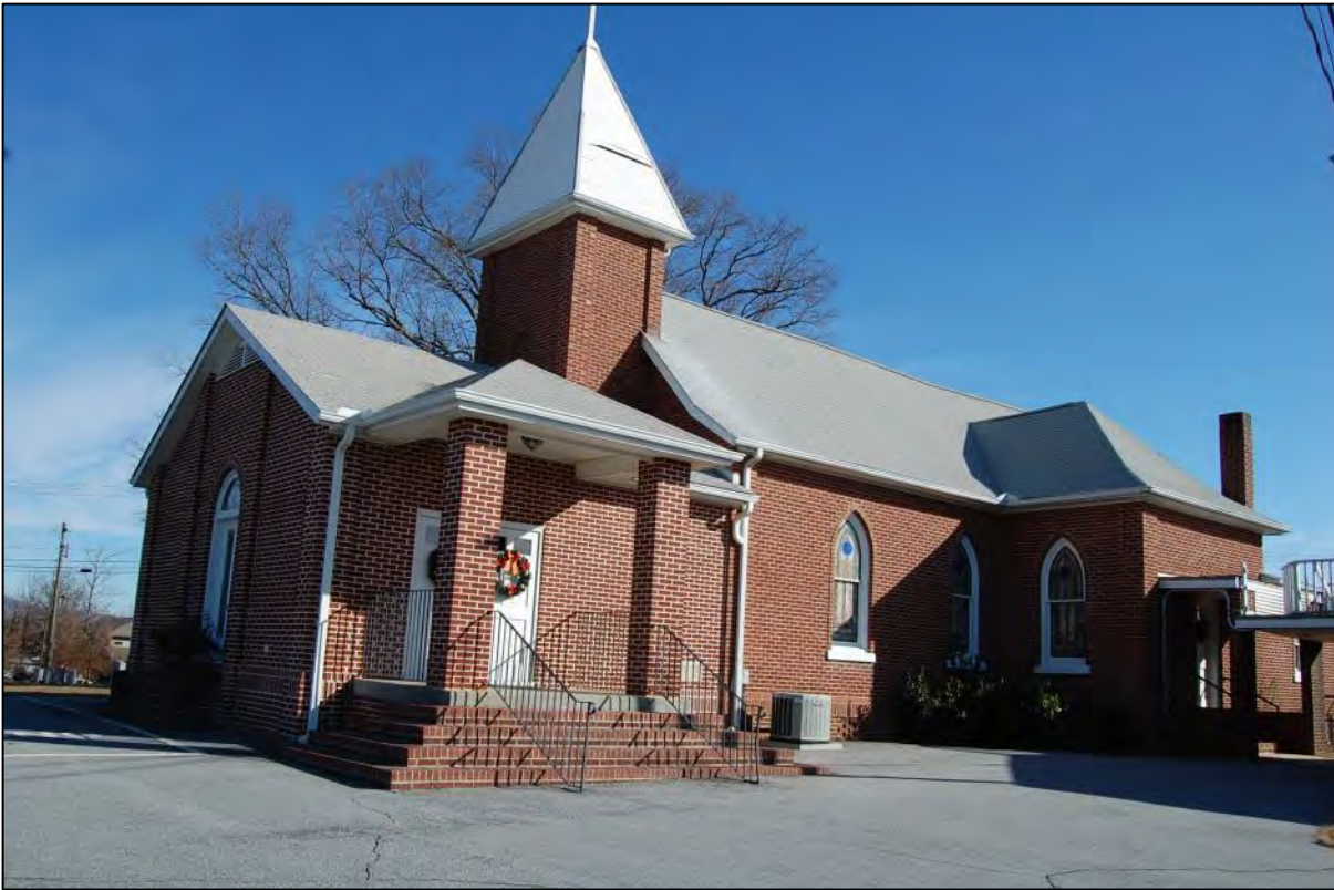
AECOM #17 – 2575 Chimney Rock Rd: W gable end and S entrance elevations
