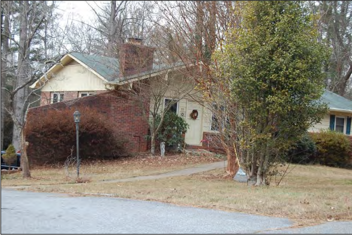
AECOM #117 - 111 Castleton Ln: E front and S side elevations
