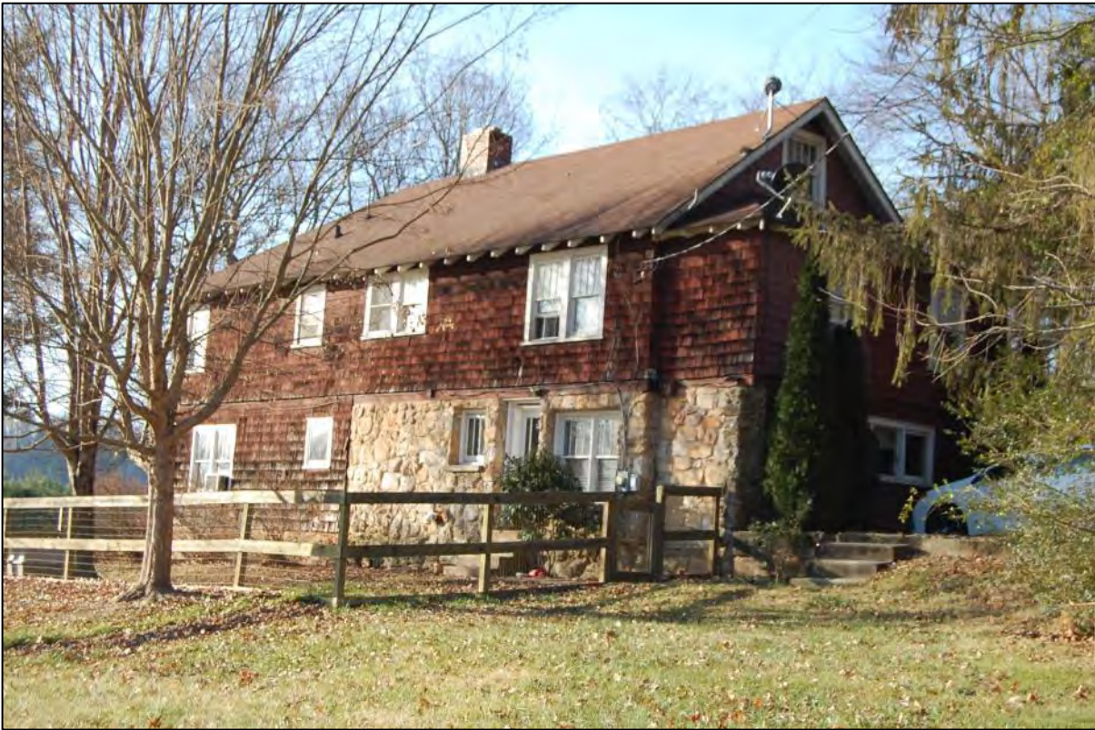
AECOM #8 - 2852 Chimney Rock Rd: N gabled and E elevations
