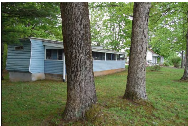
Figure 17. Looking southwest at mobile home at left and house at right
