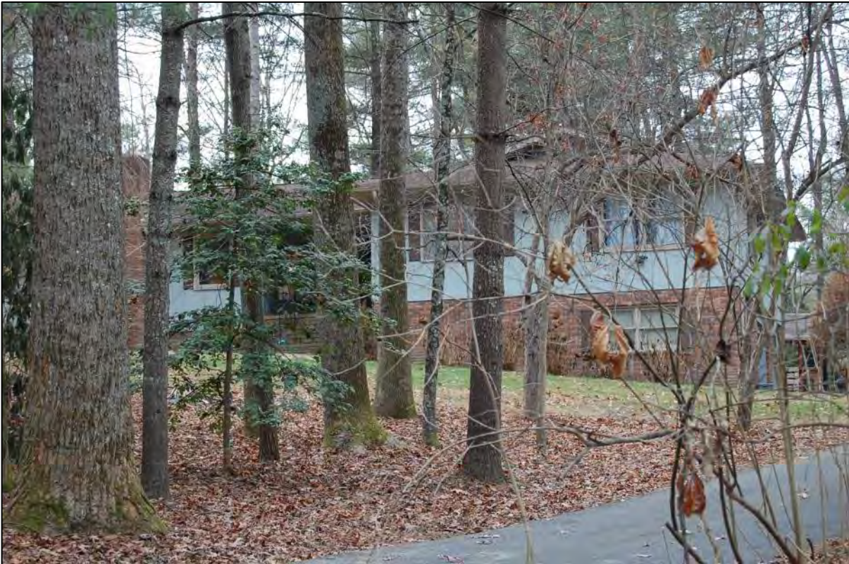
AECOM #78 - 119 Nob Hill Rd: E front and N side elevations
