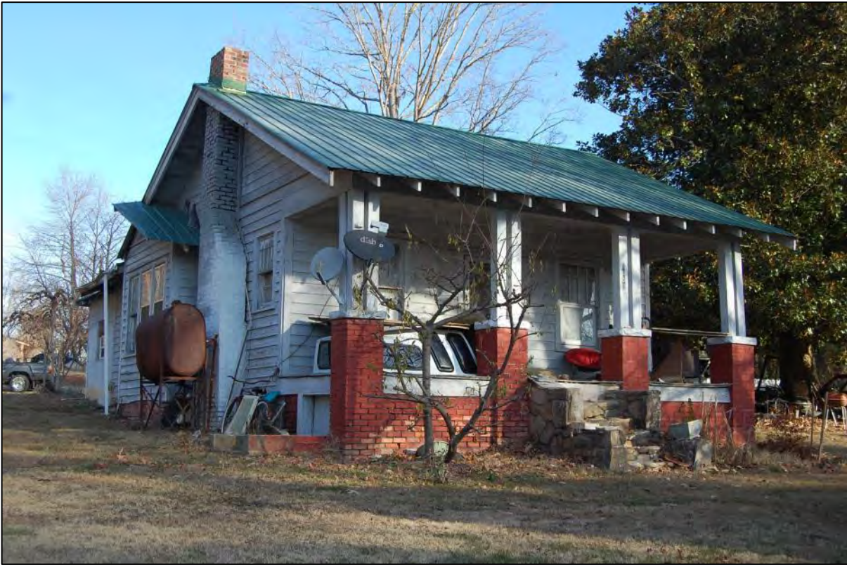
AECOM #6 - 2859 Chimney Rock Rd: S front and W side elevations
