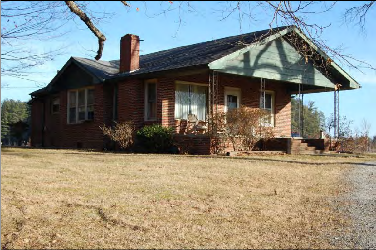
AECOM #4 - 2869 Chimney Rock Rd: S front and W side elevations
