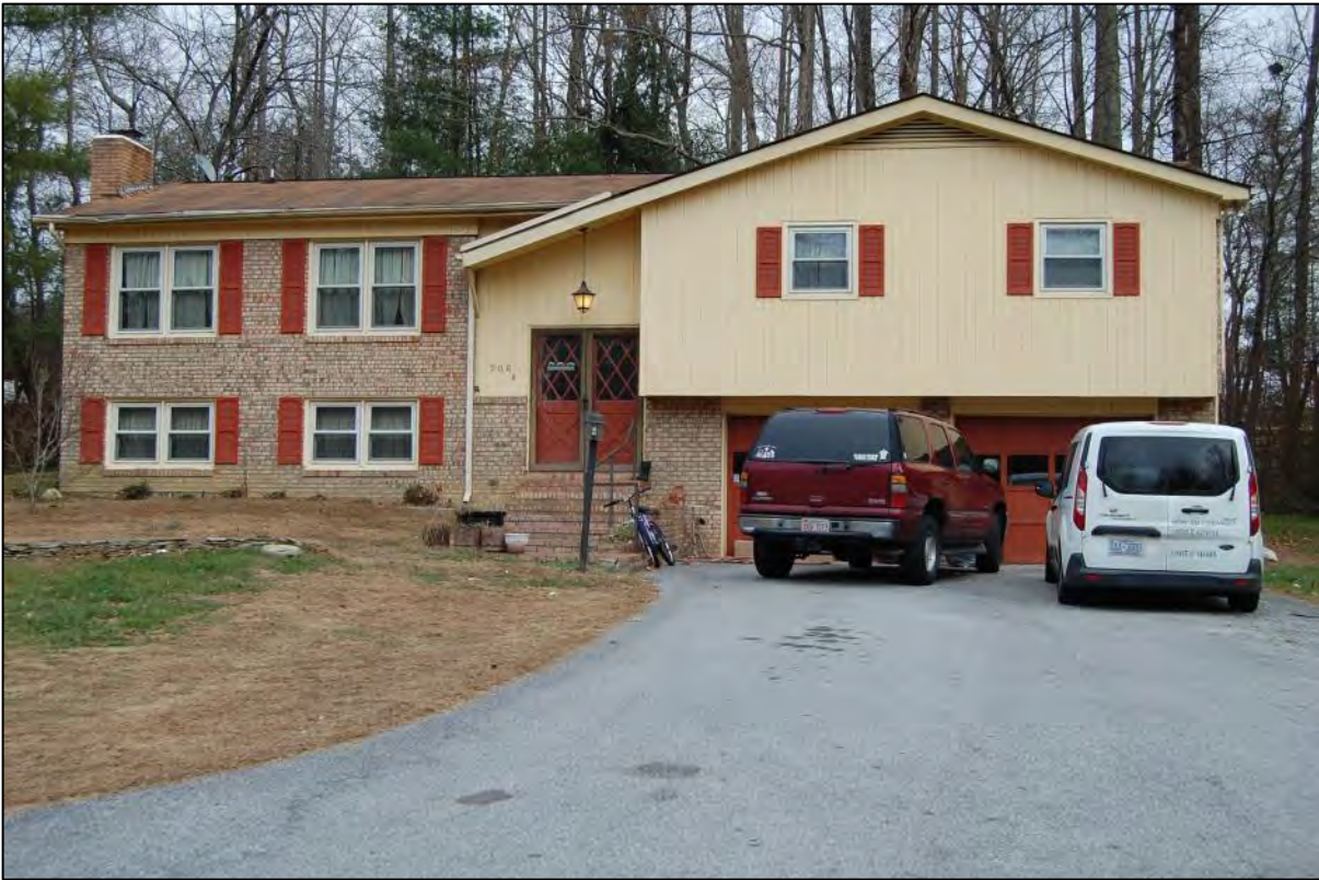
AECOM #129 - 206 Shannon Rd: W front elevation
