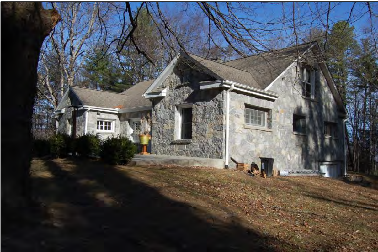
AECOM #16b - 258 St Marys Dr: SW front and SE side elevations
