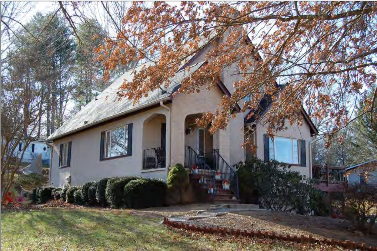
AECOM #23 - 39 Nix Rd: N front and E side elevations
