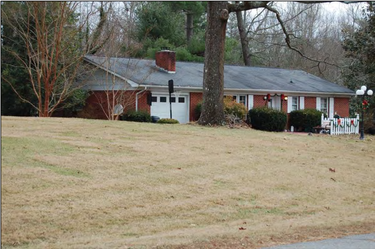
AECOM #108 - 126 Castleton Ln: W front and N side elevations
