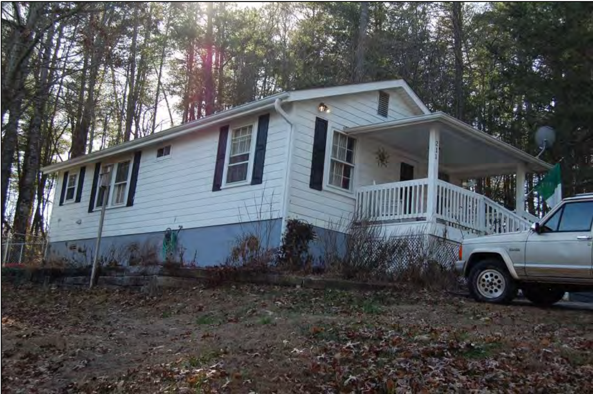
AECOM #30 - 211 Big Pine Rd: N front and E side elevations
