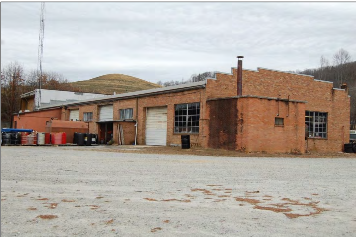
Figure 180. West and south elevations of garage with landfill rising to rear
