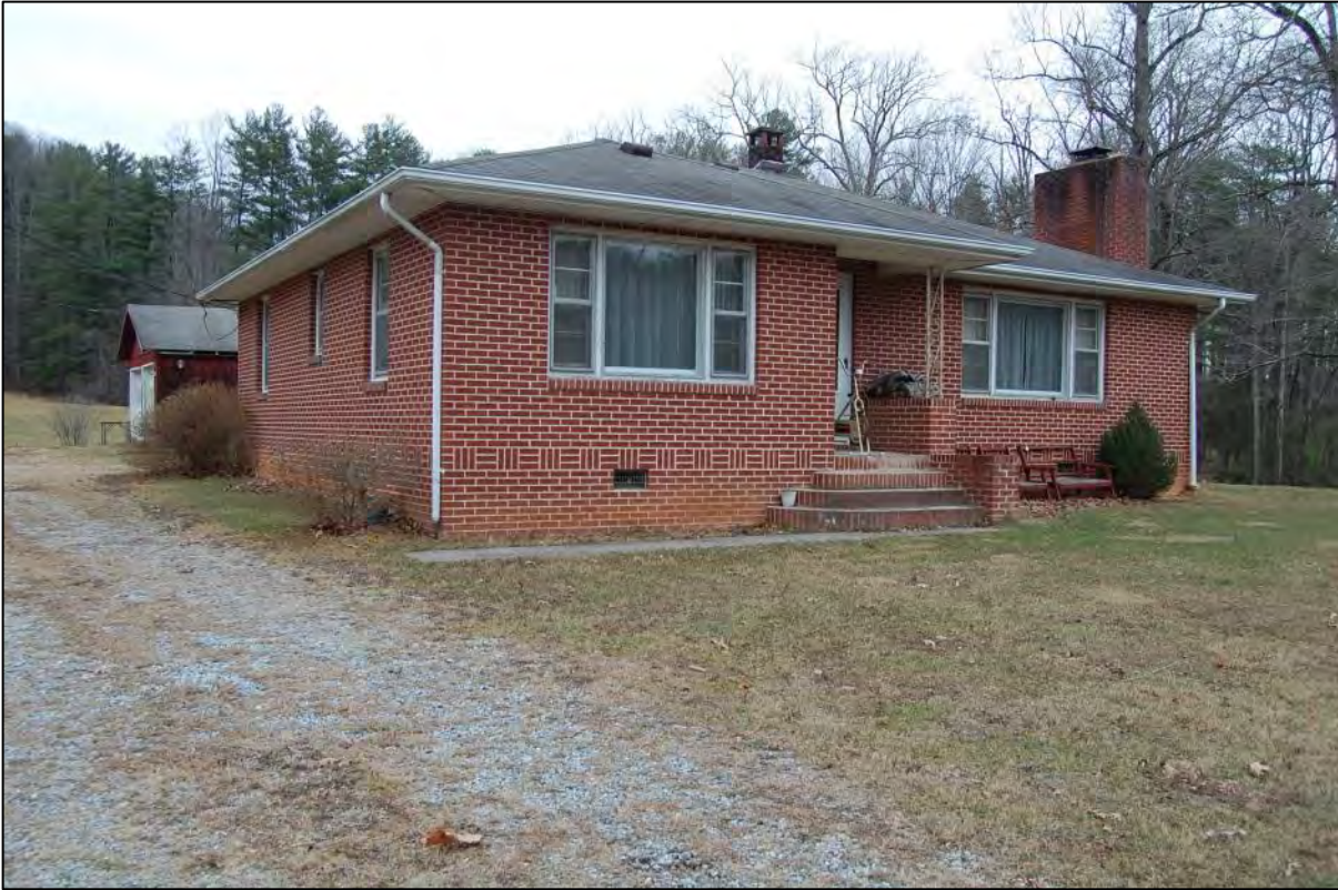
AECOM #55 - 676 Stoney Mountain Rd: SW front and NW side elevations
