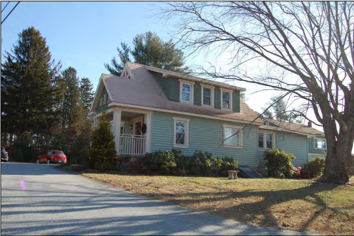
AECOM #15 - 2840 Chimney Rock Rd: N front and W side elevations of former house
