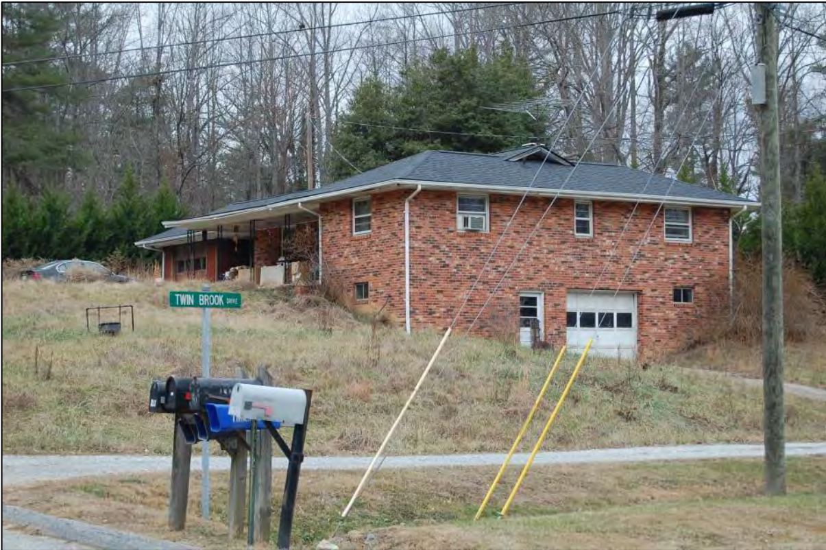
AECOM #66 - 203 Leverette Dr: S front and E side elevations
