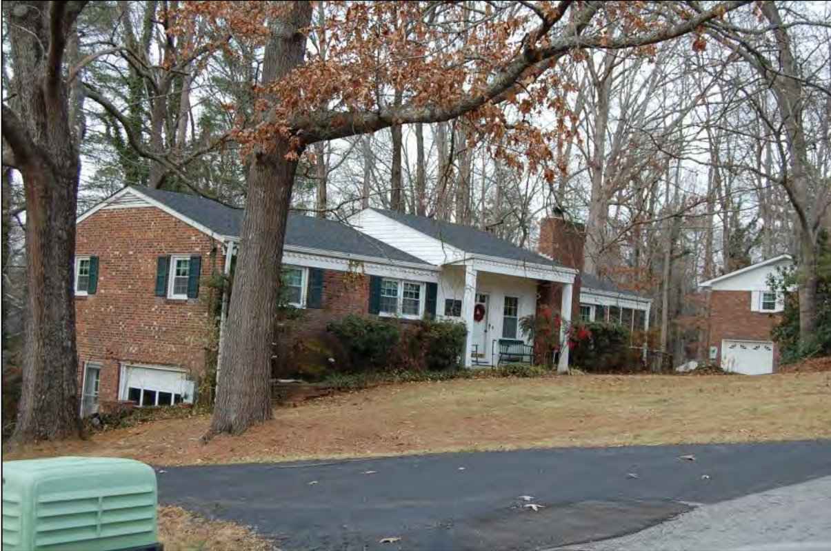
AECOM #118 - 115 Castleton Ln: E front and S side elevations
