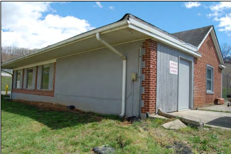
Figure 171. West side and south gable end of former washhouse
