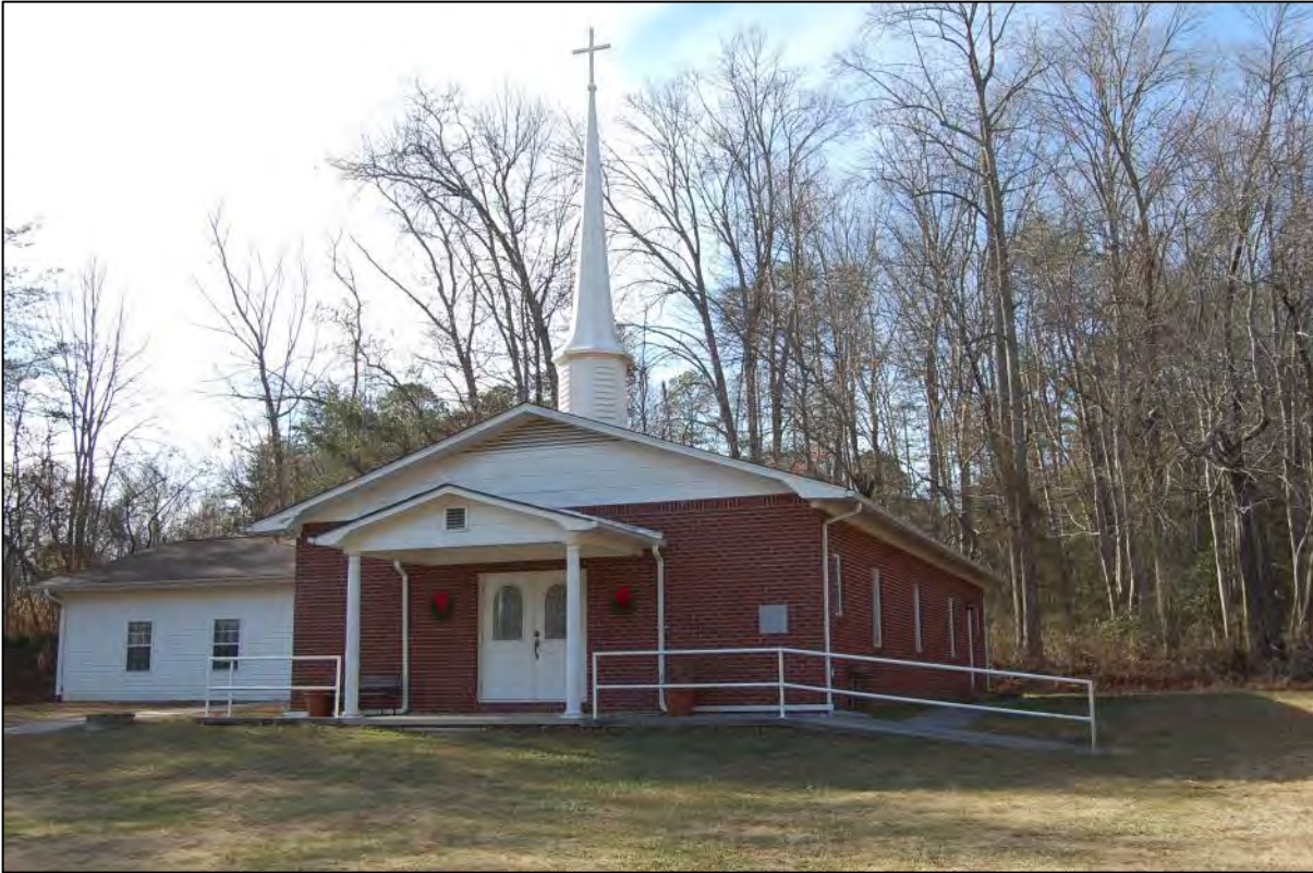
AECOM #37 - 193 Salisbury Rd: E front and N side elevations
