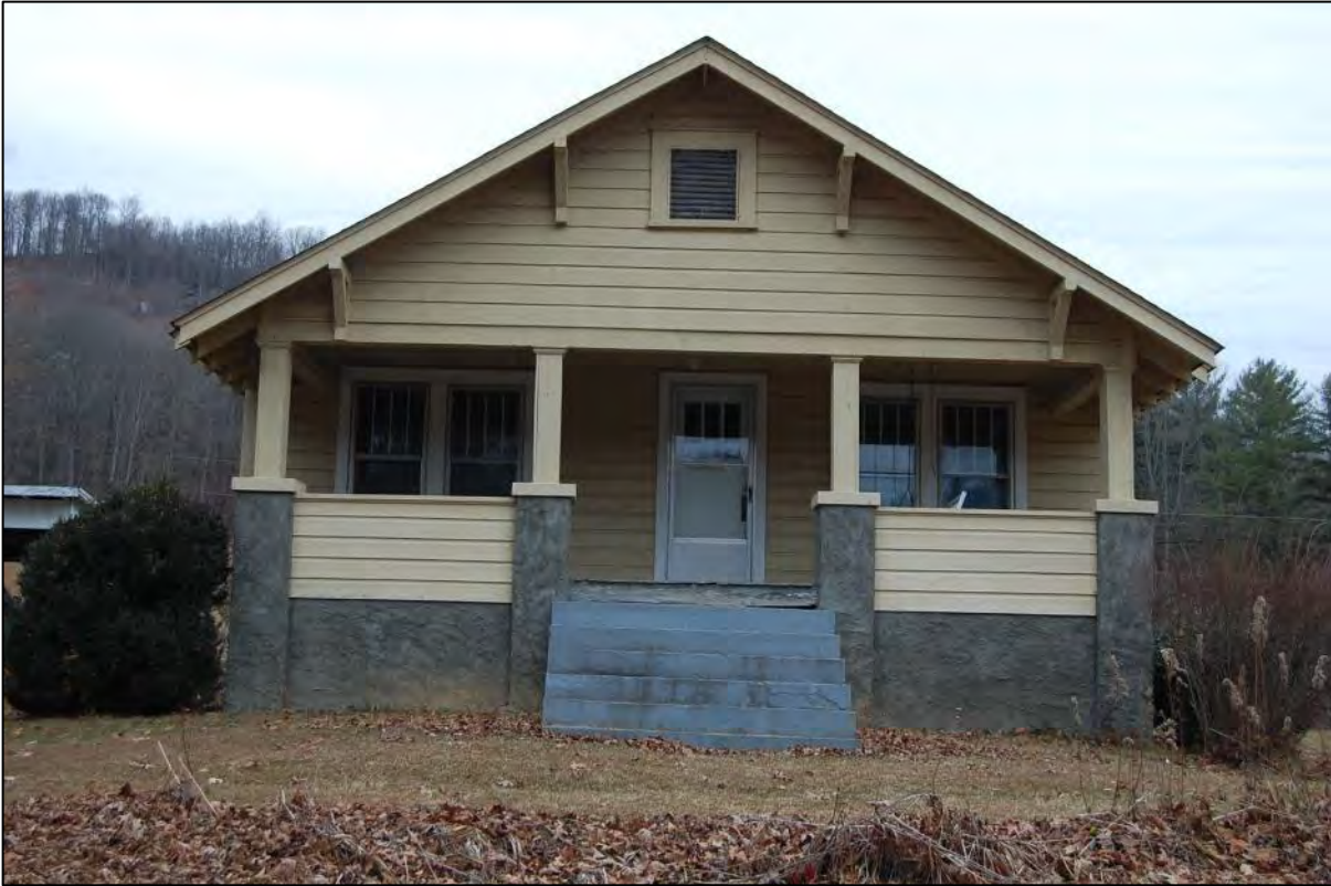
AECOM #56 - 692 Stoney Mountain Rd: SW front elevation
