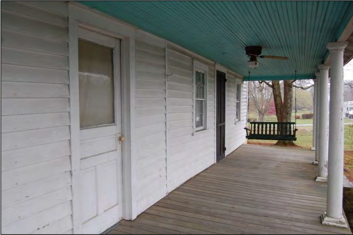
Figure 5. North front elevation with three bays of original block to right of vertical molding and later wing to left
