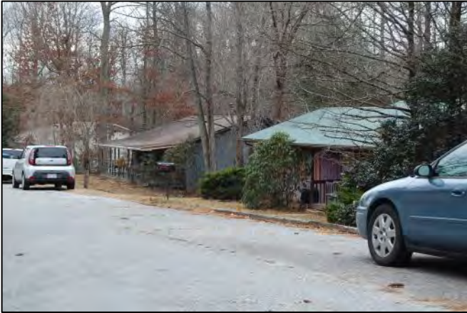
Left - Looking S down Starlight at Primrose – 38 at left (c1981) and 49 at right (c1979) Starlight Right – W side of Apple Creek S of Starlight looking SE – 25 at left (c1989), 27 at center (c1980), 29 Apple Creek at right (c1982)
