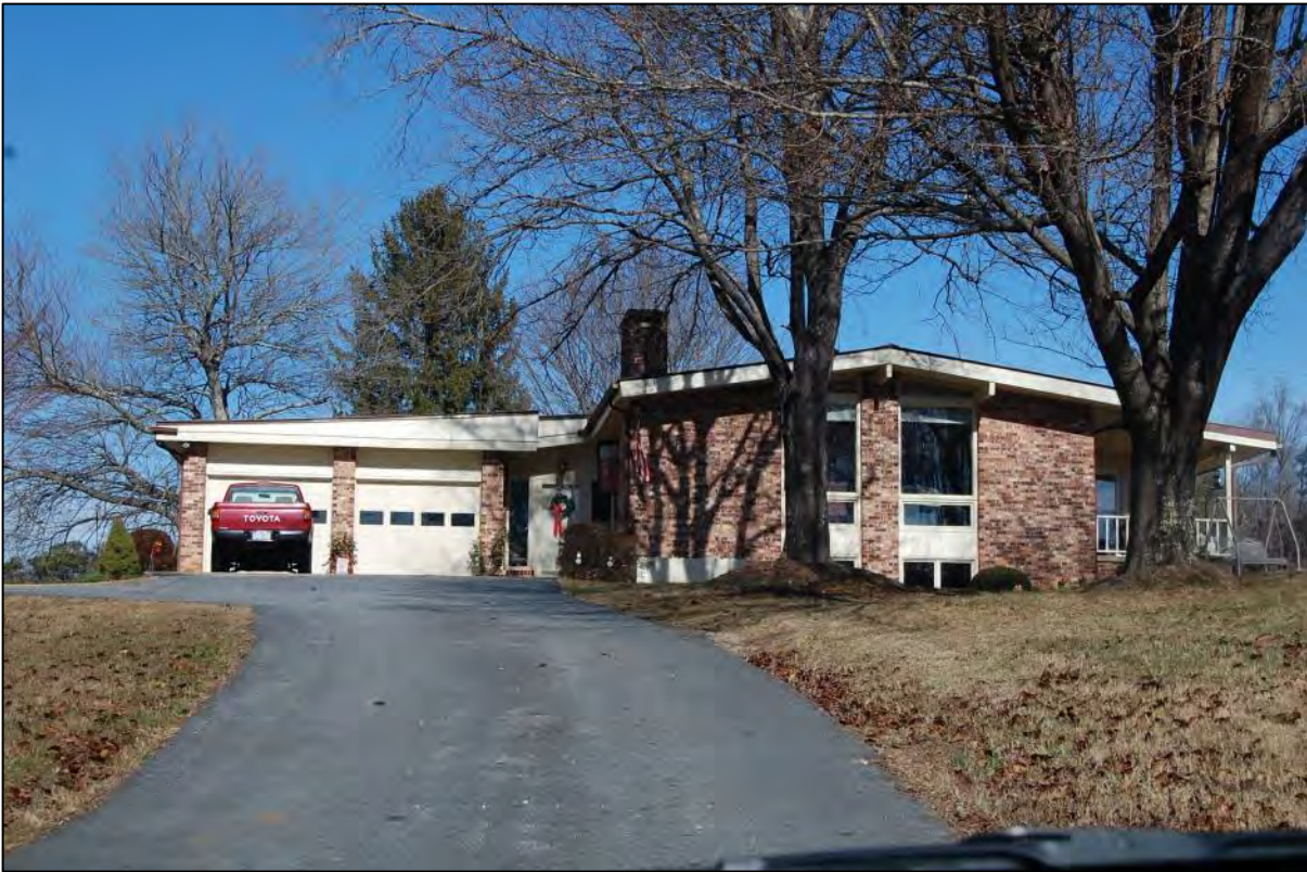
AECOM #25 - 168 Nix Rd: S front and W side elevations
