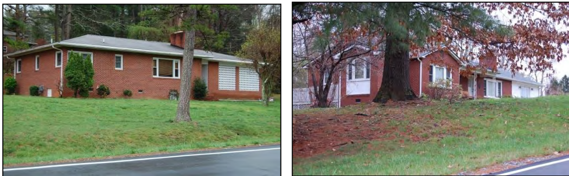
Figure 104. 102 Brookside Camp Road at left and 3228 Florida Drive at right
