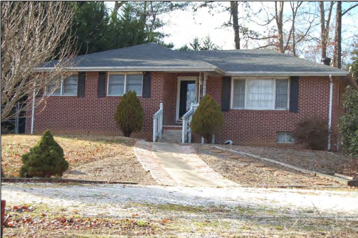
AECOM #40 - 509 Brookside Camp Rd: E front and N side elevations
