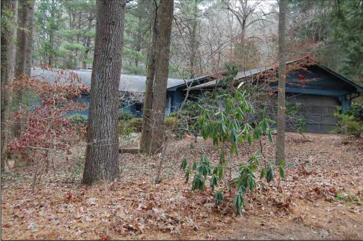
AECOM #87 - 116 Nob Hill Rd: W front and N side elevations
