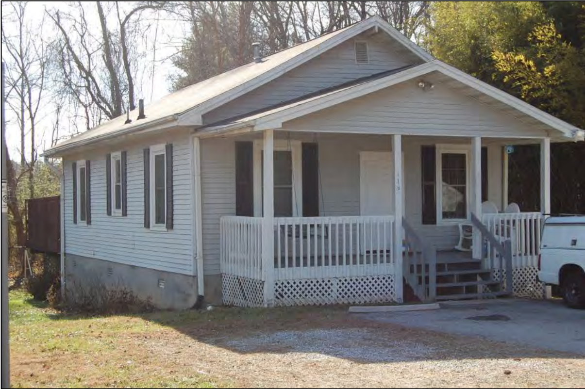
AECOM #27 - 115 Big Pine Rd: N front and E side elevations
