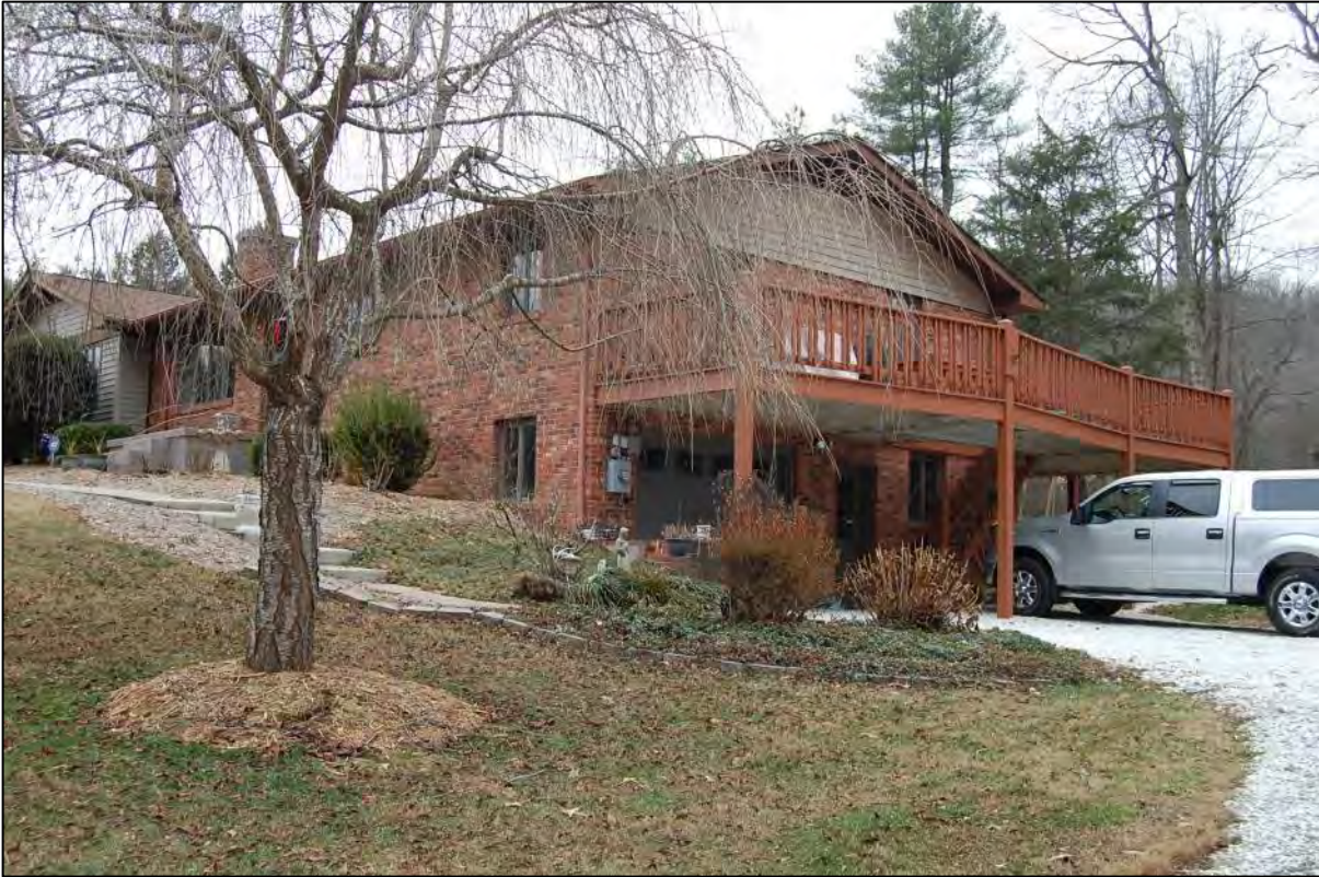
AECOM #67 - 109 Twin Brook Dr: E front and N side elevations
