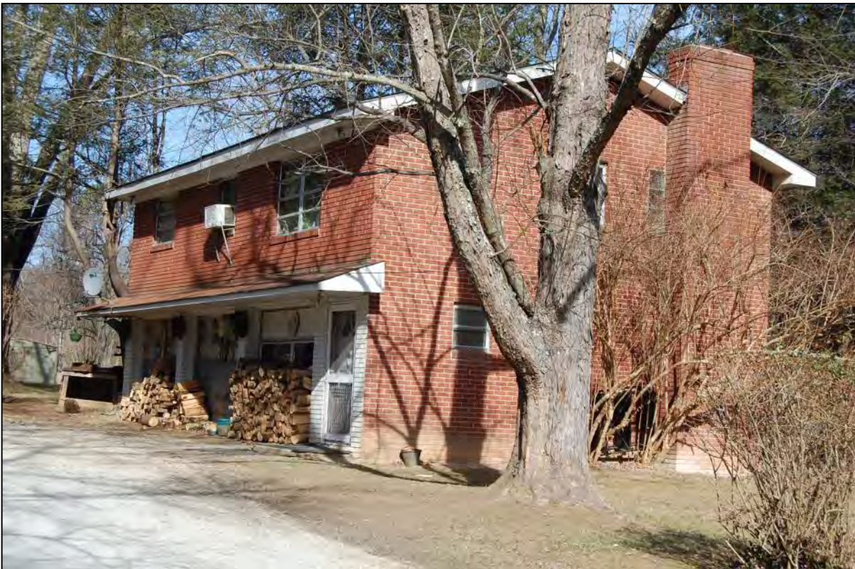
AECOM #26 - 51 Old Holbert Rd: W front and S side elevations of garage/apartment
