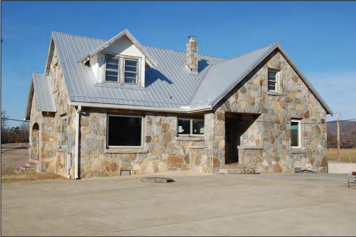
AECOM #13 - 384 Suitland Rd: long E and gable-end S elevations
