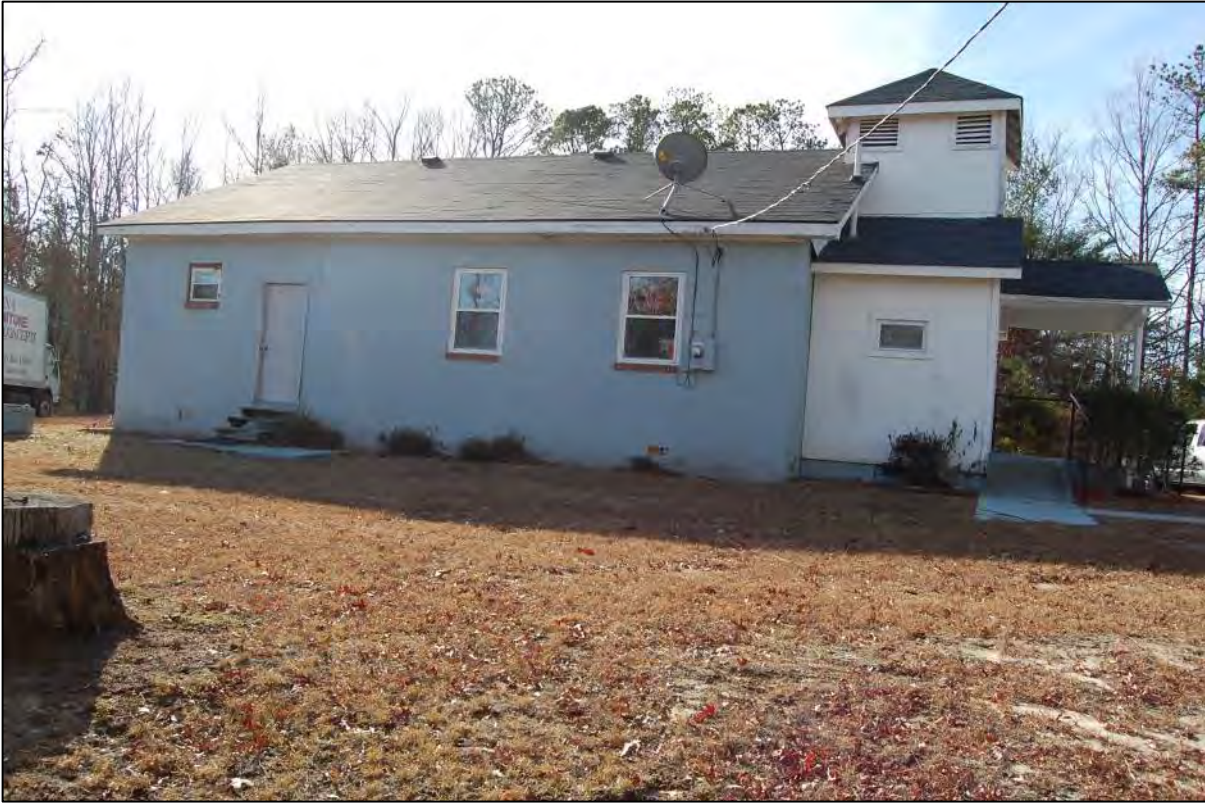
AECOM #36 - 314 N Clear Creek Rd: E side elevation
