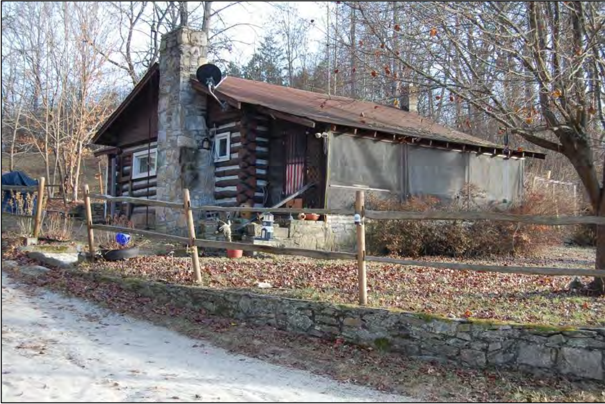
AECOM #52 - 239 Balfour Rd: W front and N side elevations
