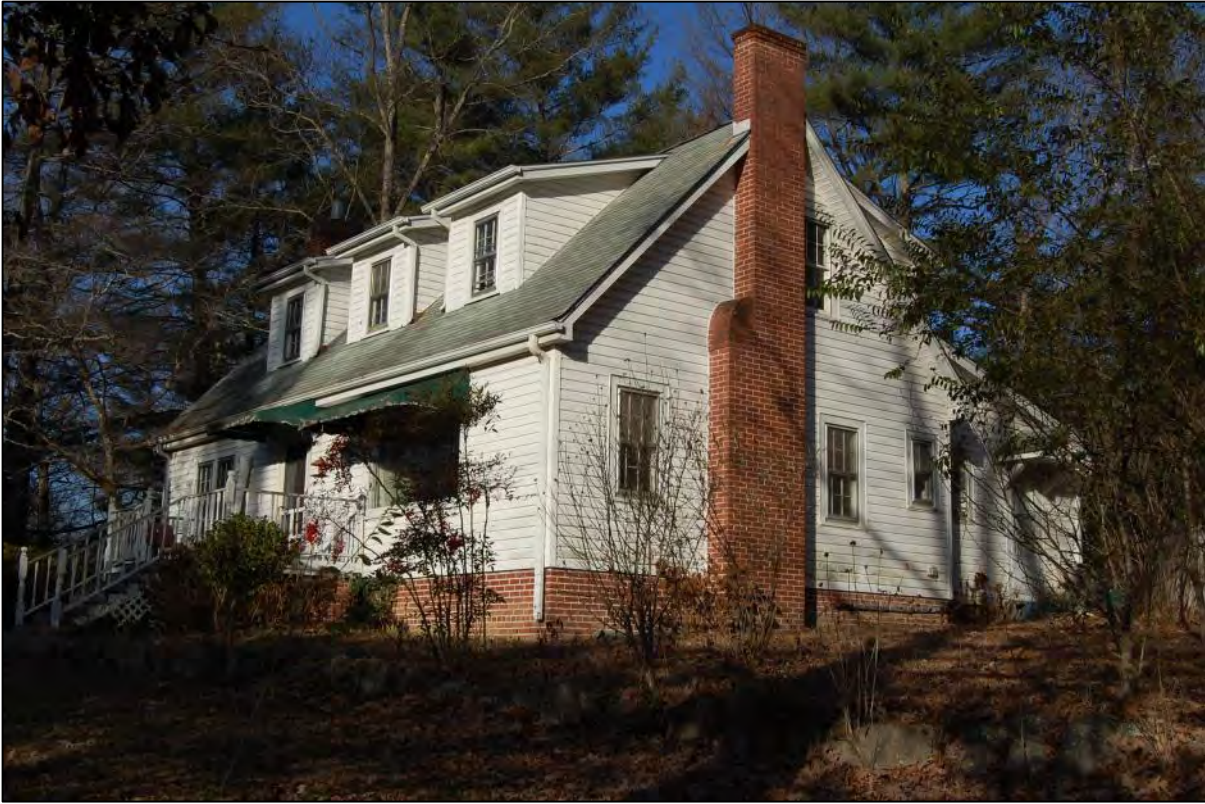
AECOM #7 - 2853 Chimney Rock Rd: S front and E side elevations
