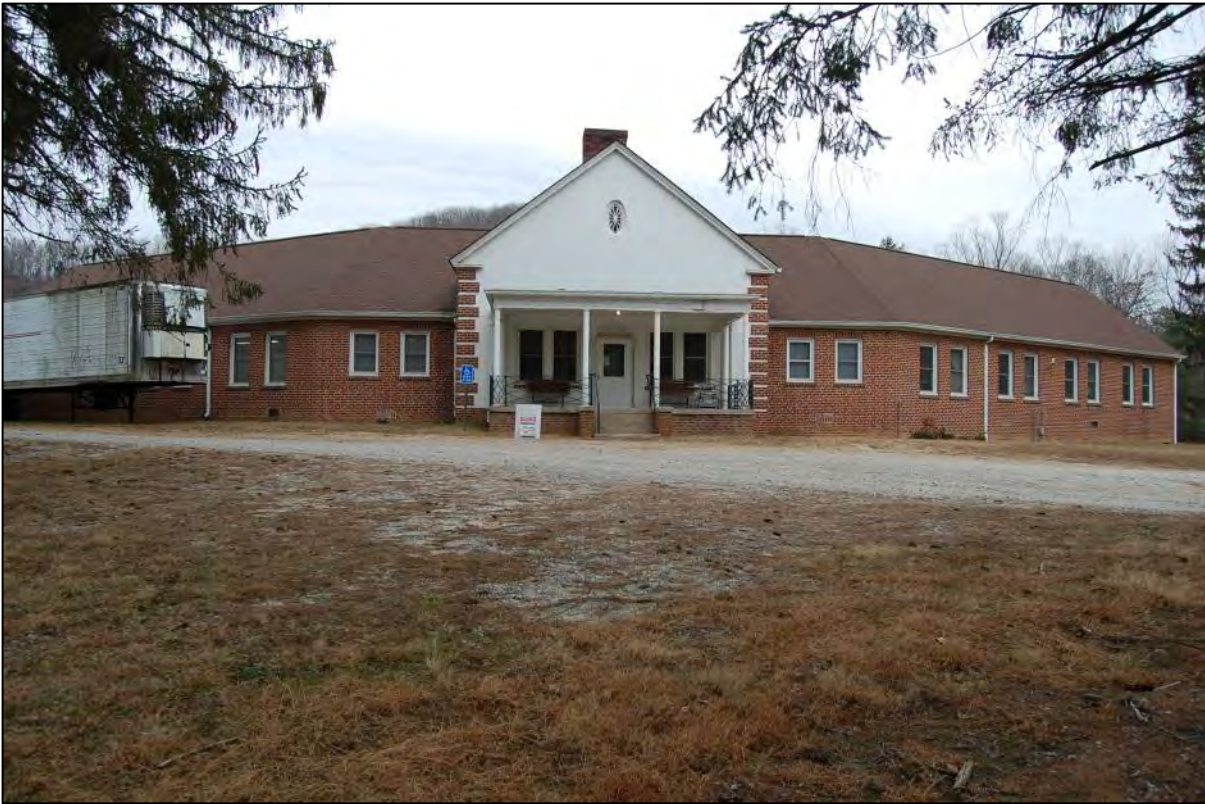
AECOM #58 – 800 Stoney Mountain Rd: W front elevation
