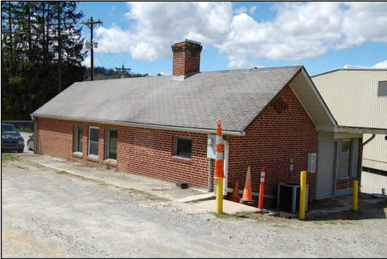
Figure 170. East side and north gable end of former washhouse
