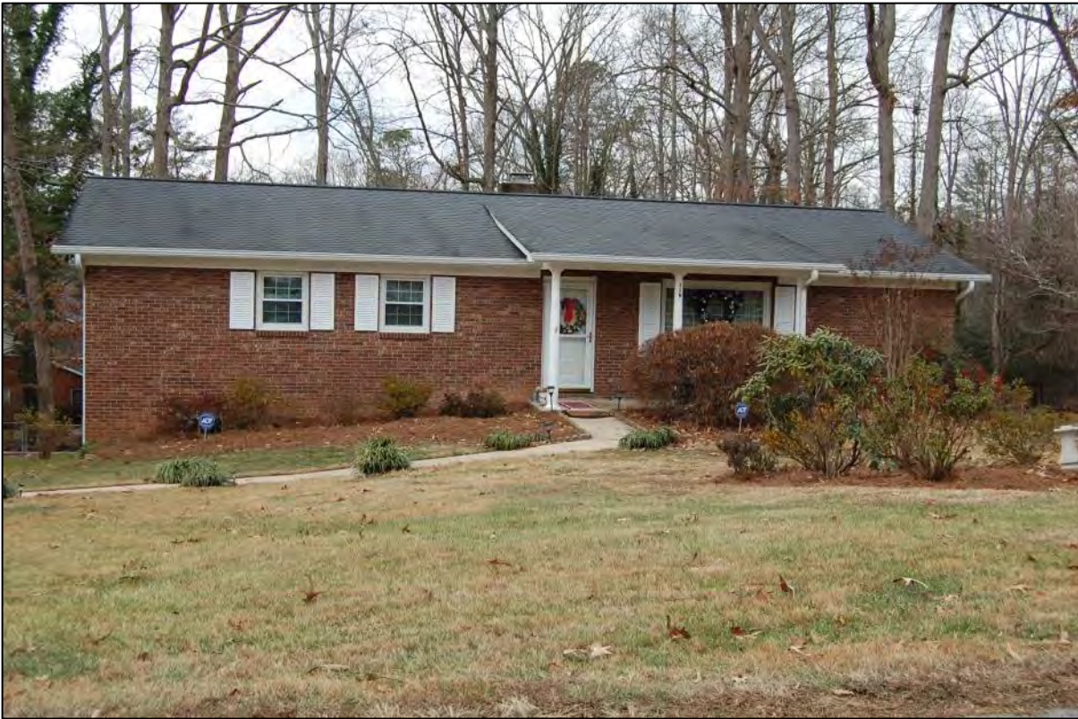
AECOM #119 - 119 Castleton Ln: E front elevation
