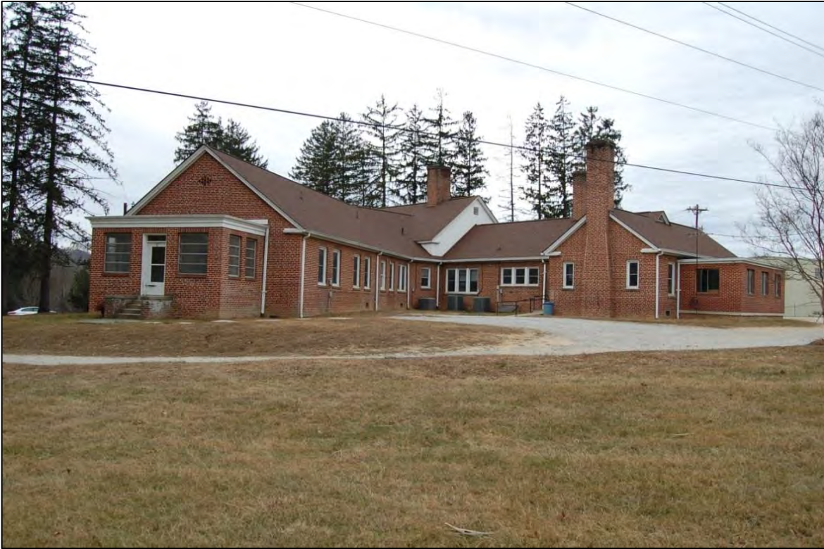
Figure 166. Looking northwest at side and rear of former residential block’s southern wing, to left, and south side of rear service ell and superintendent’s wing, at right
