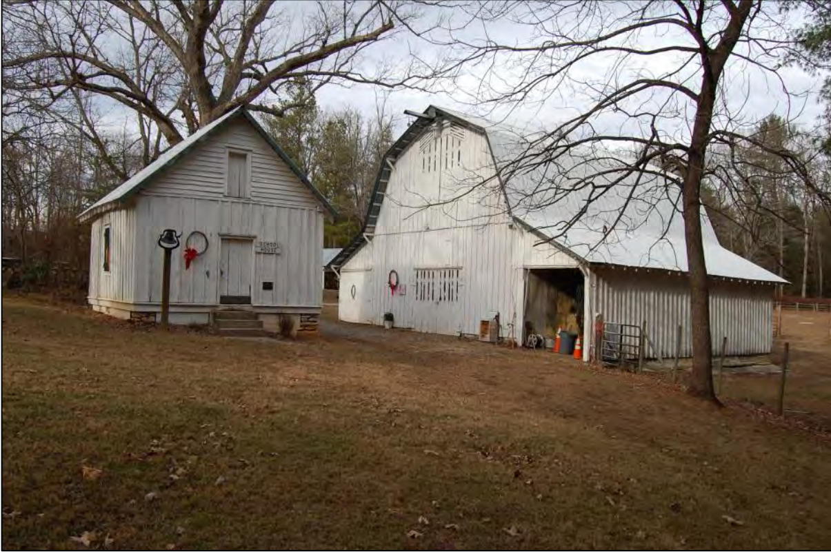
AECOM #135 (HN0043) - 3346 Haywood Rd: View looking NE at schoolhouse (moved to property) and barn (1923)
