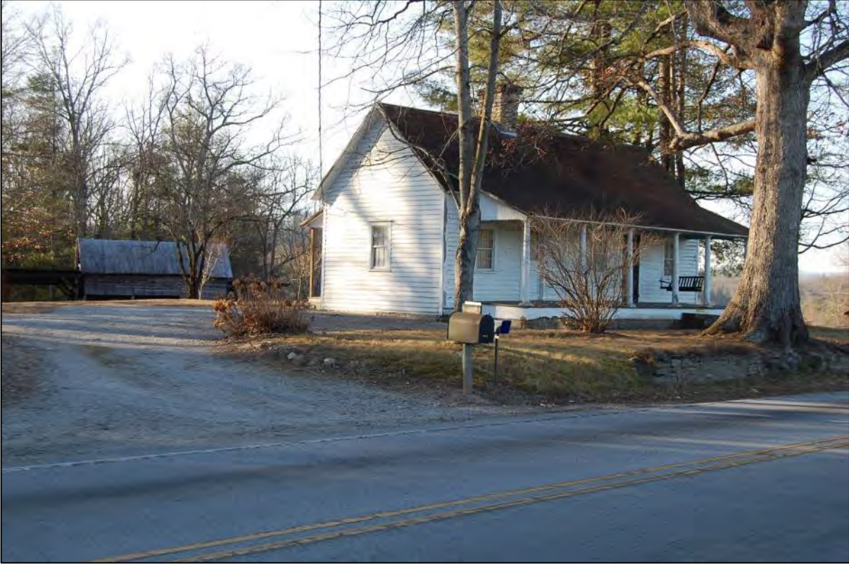
AECOM #3/HN1355 - 2886 Chimney Rock Rd: N front and E side elevations; barn at left distance
