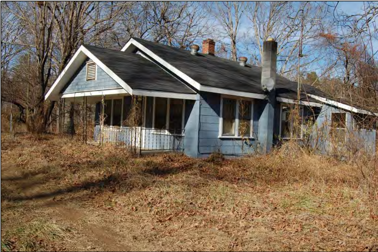
AECOM #34 - 2791 Howard Gap Rd: SW front and SE side elevations
