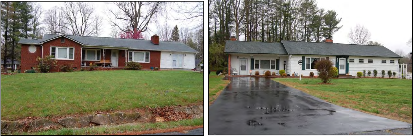
Figure 94. 3228 Florida Drive (left) and 3159 Cheryl Drive (right) with side additions
