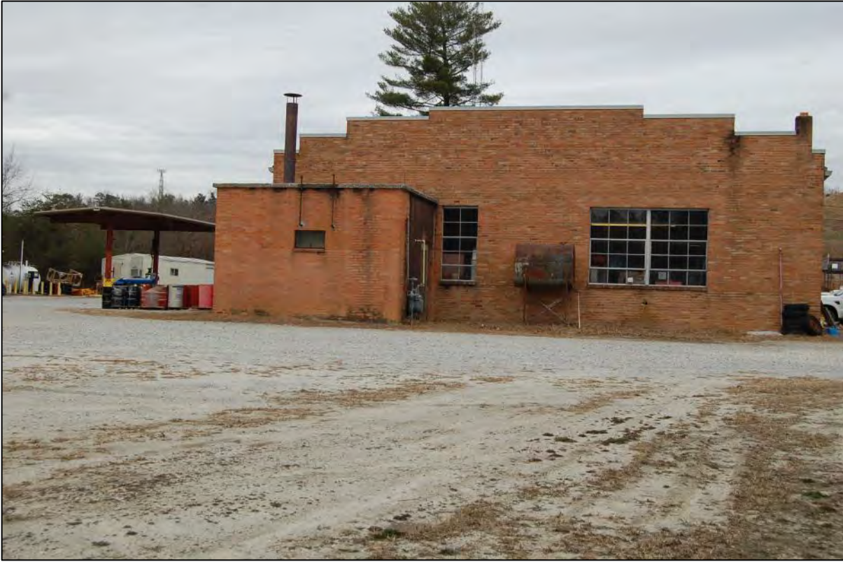
AECOM #59 - 812 Stoney Mountain Rd: S front elevation
