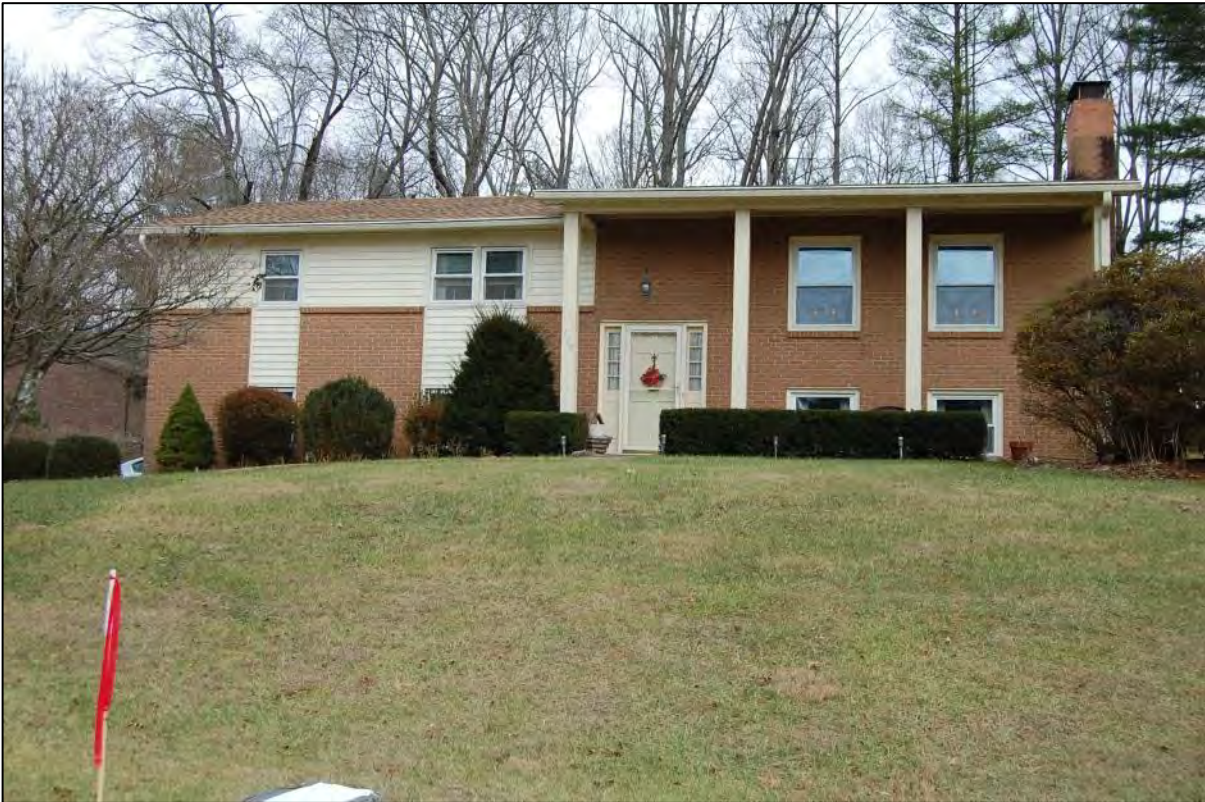
AECOM #132 - 108 Shannon Rd: W front elevation
