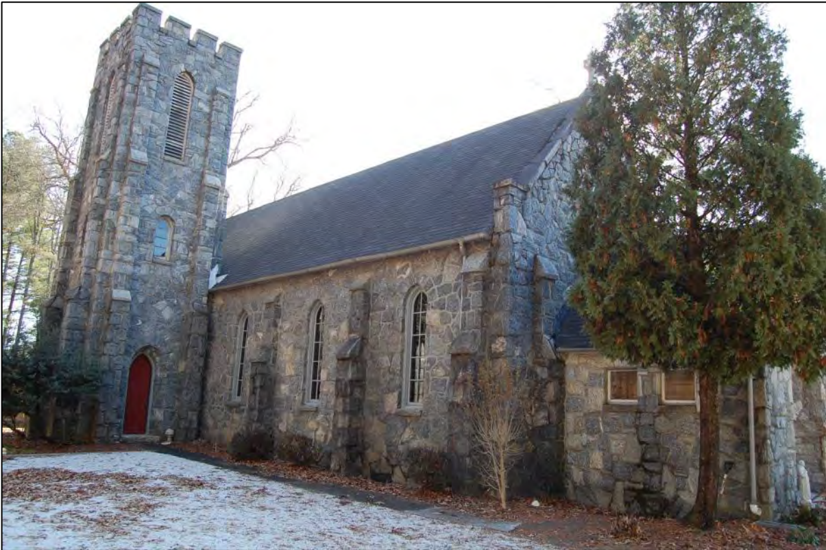
AECOM #16a - 186 St Marys Dr: N side and W front elevation of church
