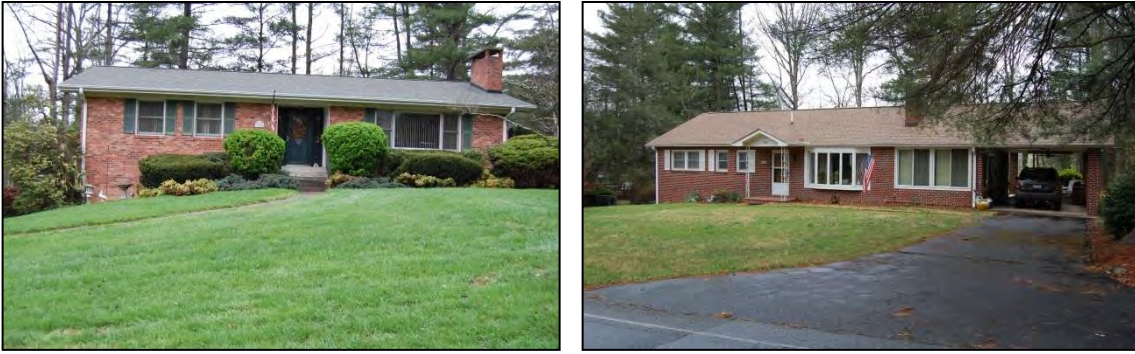
Figure 97. 3210 Cardinal Lane at left and 3160 Cardinal Lane at right
