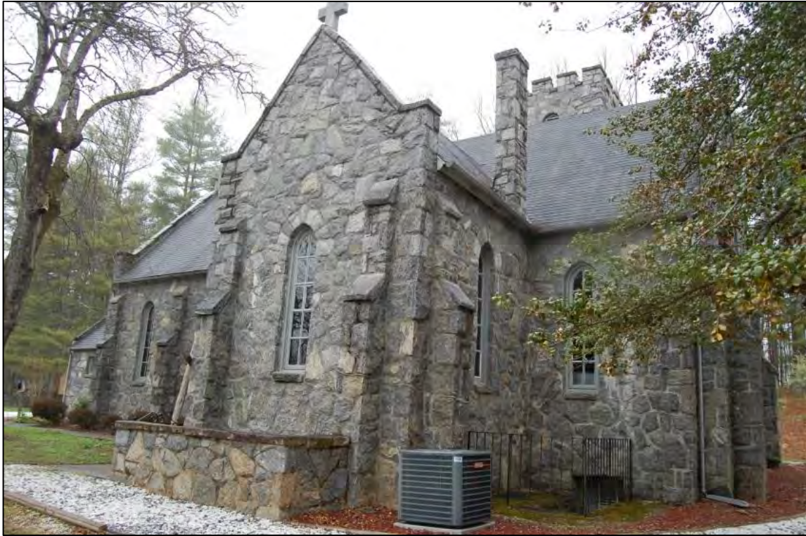
Figure 28. South side and east rear elevations of St. Mary's Chapel
