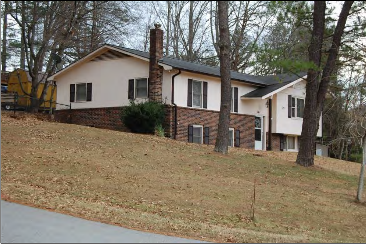
AECOM #133 - 100 Shannon Rd: W front and N side elevations
