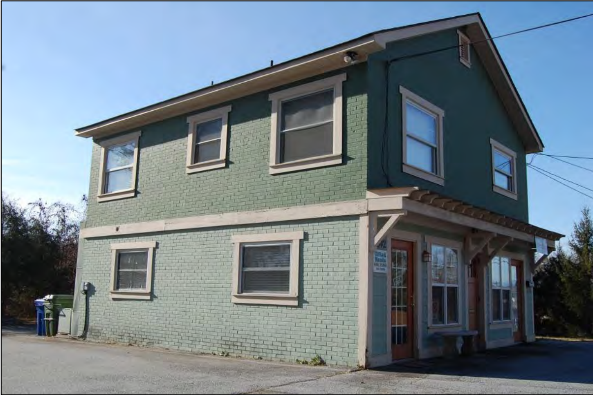
AECOM #15 - 2840 Chimney Rock Rd: E side and S rear elevations of former garage
