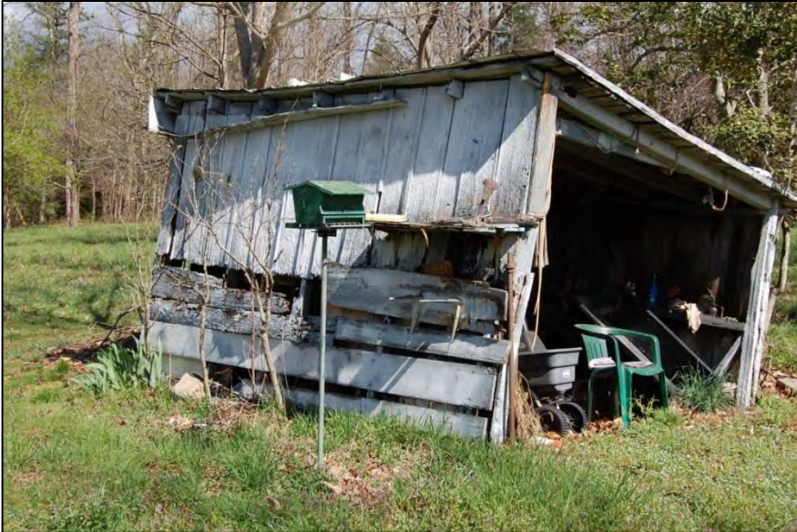
Figure 216. Southwest and southeast (open) elevations of tool house
