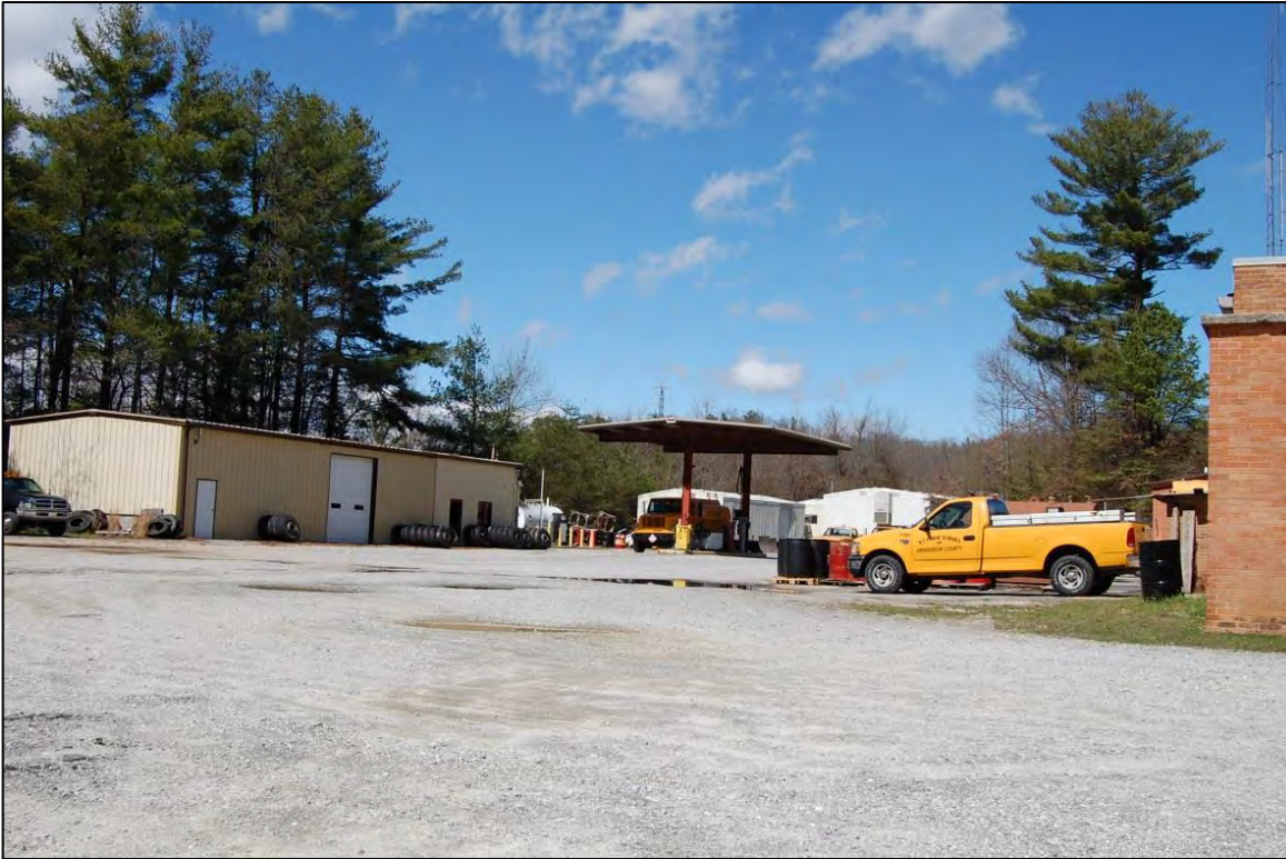
Figure 183. Looking northwest at metal storage building, at left, fuel pump canopy, at center, and corner of garage, at far right
