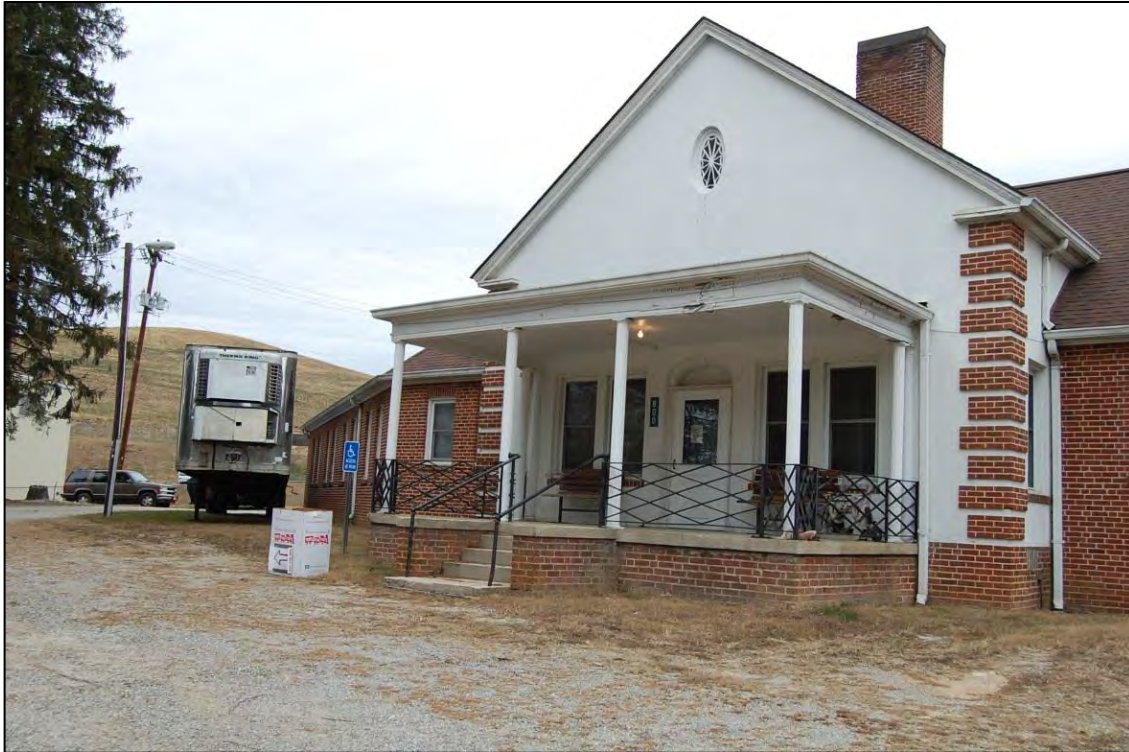
Figure 164. Looking northeast at former residential block’s principal entry and northern wing
