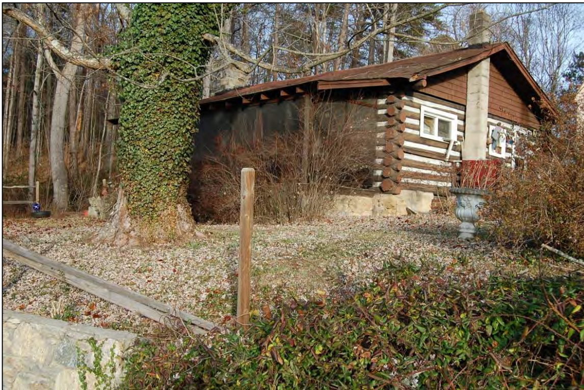
Figure 76. West front and south side elevations of house; note retaining wall along road at left foreground
