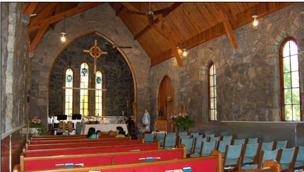
Figure 31. St. Mary's Chapel looking southeast toward chancel; note dark stone between bays at right (south) from first construction period
