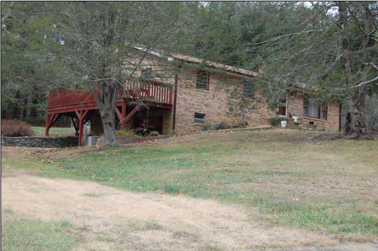
AECOM #68 - 208 Leverette Dr: E side and N front elevations
