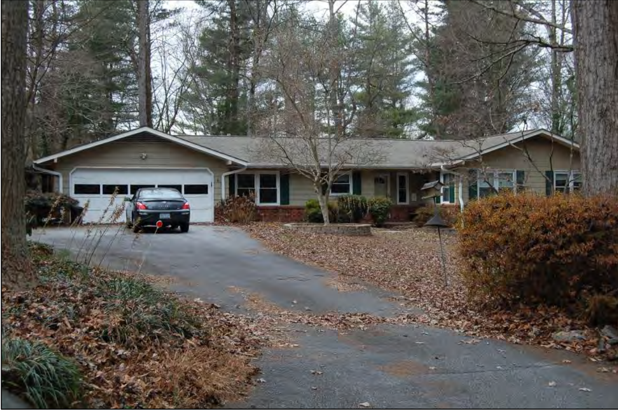
AECOM #77 - 115 Nob Hill Rd: E front elevation
