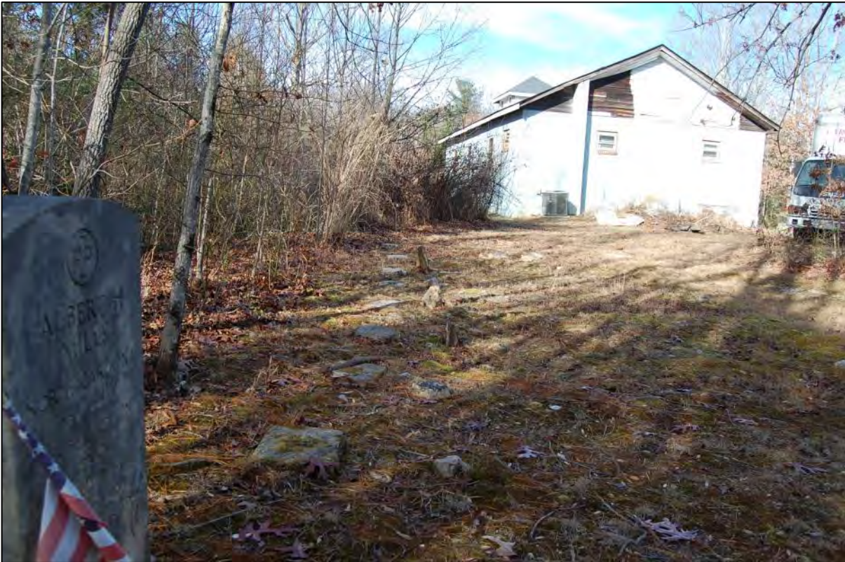
AECOM #36 - 314 N Clear Creek Rd: cemetery in foreground, S rear and W side elevations of church at right
