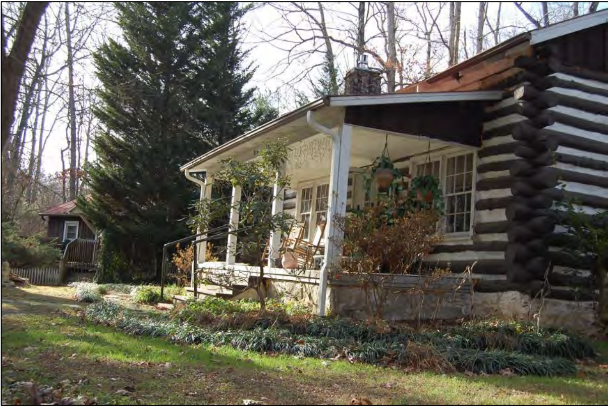
AECOM #41 - 515 Brookside Camp Rd: S front and E side elevations of log cabin; frame cabin at left
