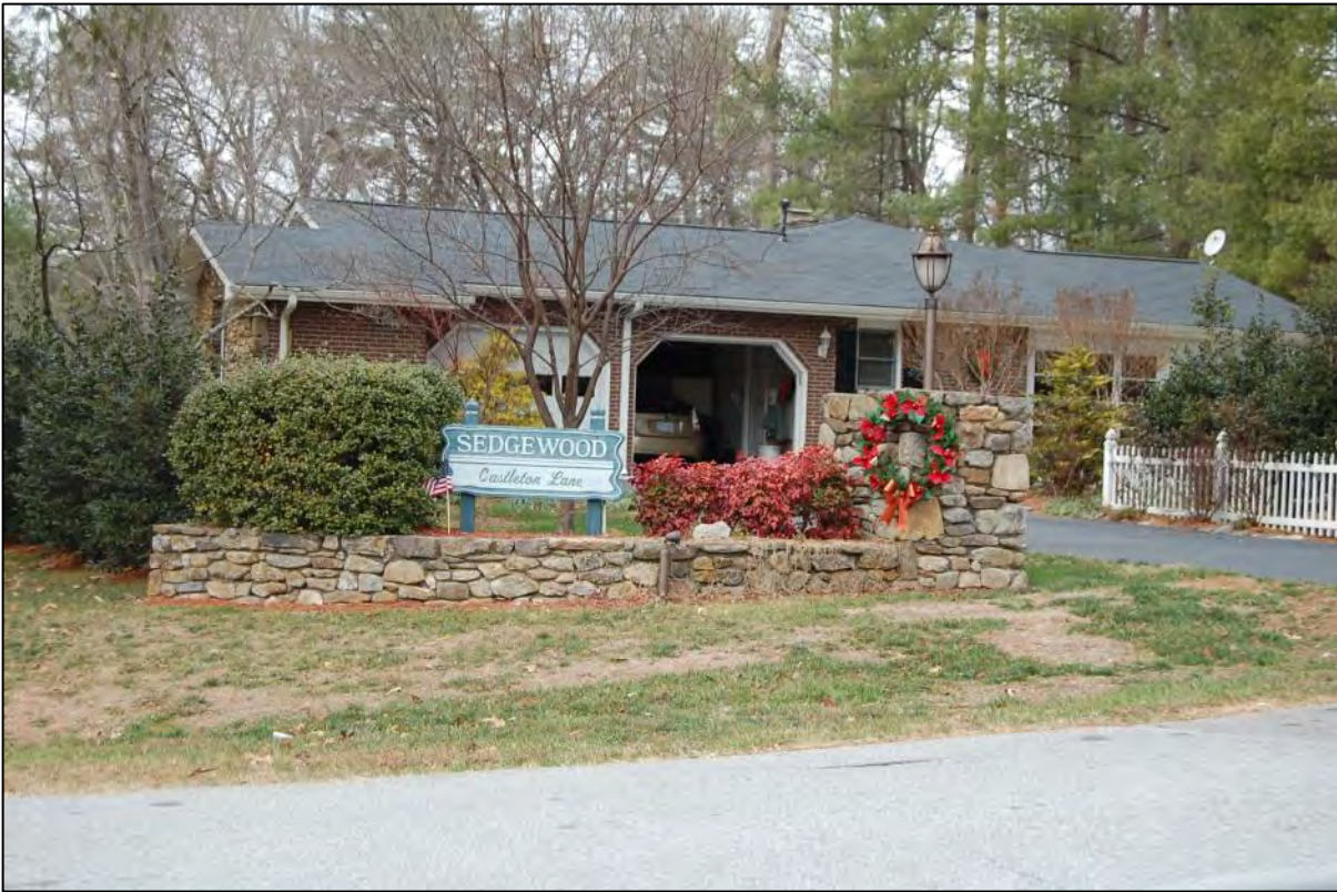
AECOM #115 - 103 Castleton Ln: E front and S side elevations
