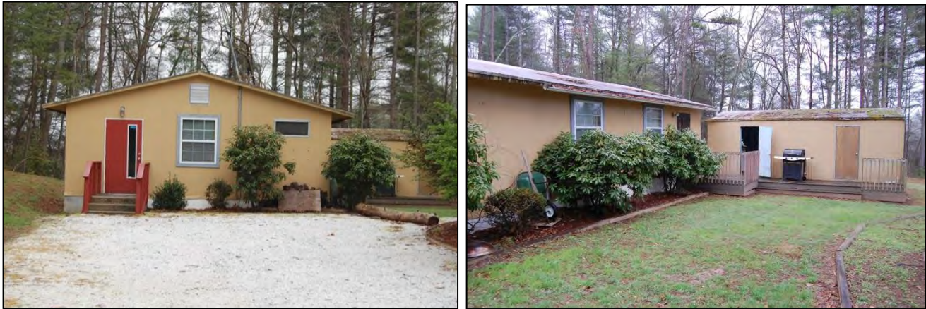
Figure 36. Looking east at office and shed, at left, and northeast, at right
