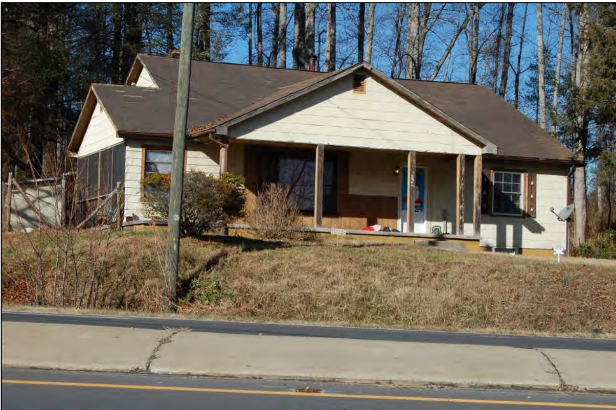
AECOM #19 - 2627 Chimney Rock Rd: SE front and SW side elevations
