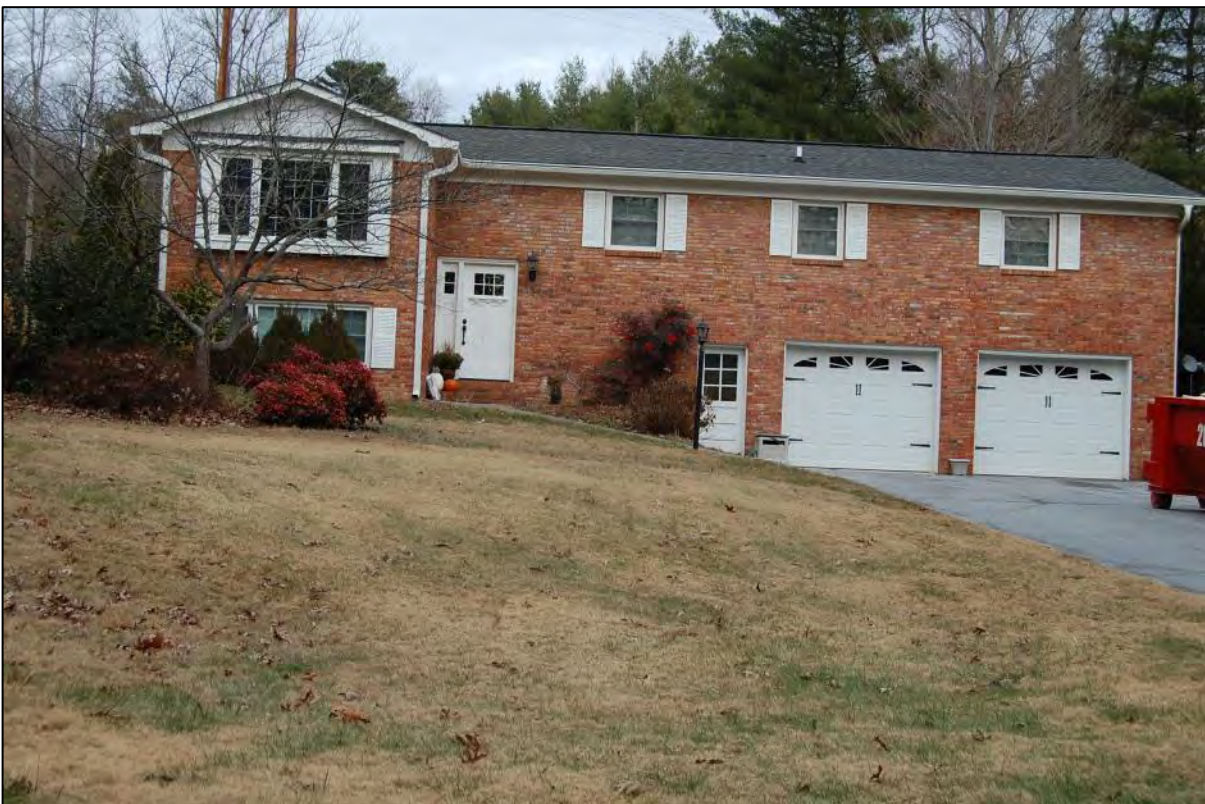
AECOM #124 - 226 Shannon Rd: SW front elevation
