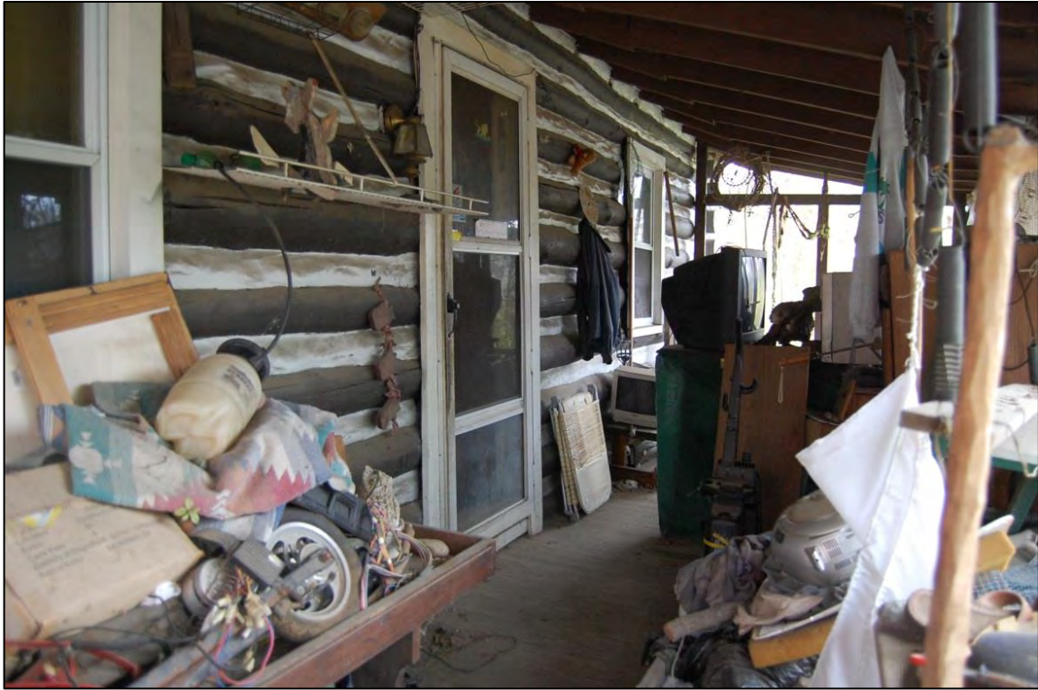
Figure 77. Front elevation of house; note scarf joints at rafters
