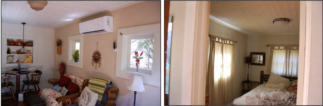
Figure 64. Northeast windows of frame house's living room, at left; looking south into bedroom from living room, at right
