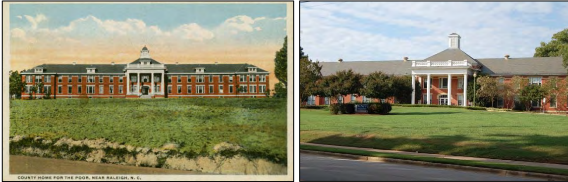
Figure 174. Postcard of Wake County Home, built 1913-1914, at left (source: North Carolina Postcards, UNC-CH); former home, now Monarch Community Health, 2017
