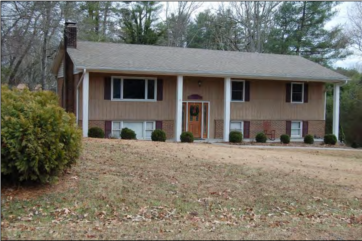
AECOM #112 - 110 Castleton Ln: W front and N side elevations
