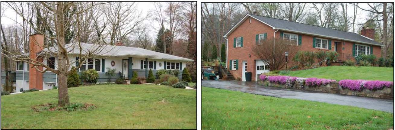
Figure 91. 3107 Florida Drive (left) and 3123 Cheryl Drive (right) are Ranch houses with the addition of a basement level holding a garage, typical of the Raised Ranch typology
