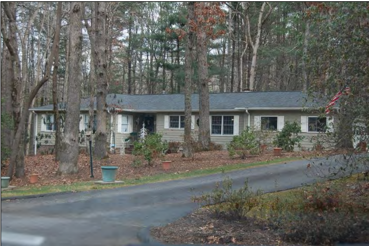
AECOM #84 - 16 Colonial Way: W front and S side elevations
