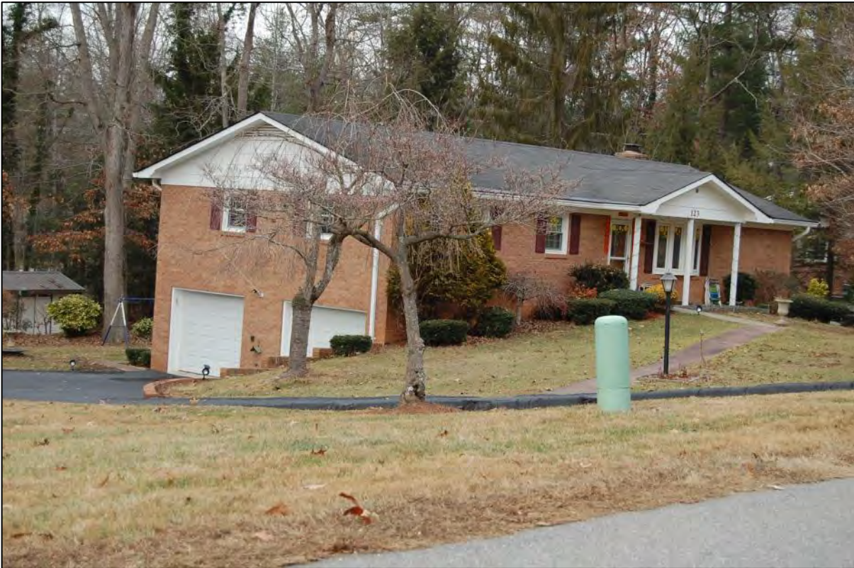
AECOM #120 - 123 Castleton Ln: E front and S side elevations
