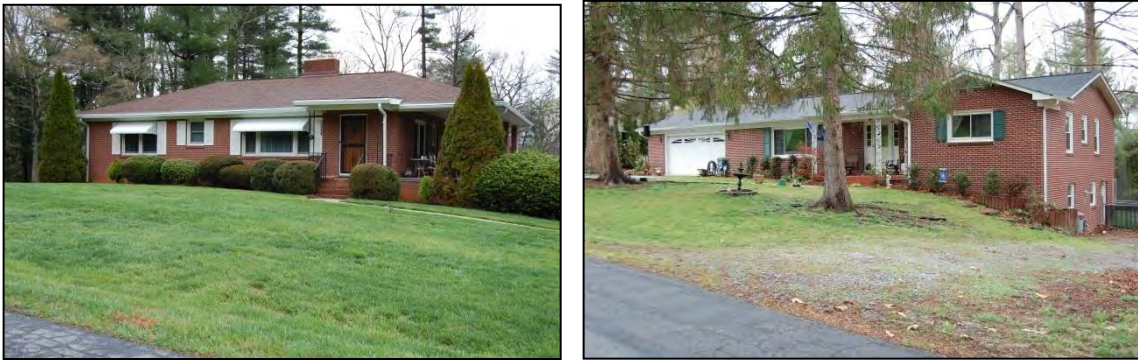
Figure 98. 3150 Cardinal Lane at left and 3140 Cardinal Lane at right
