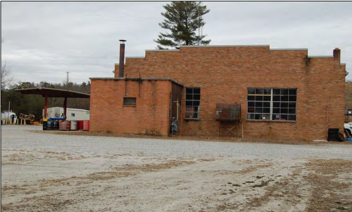
Figure 179. South elevation of garage; note open metal canopy over gas pumps, at left
