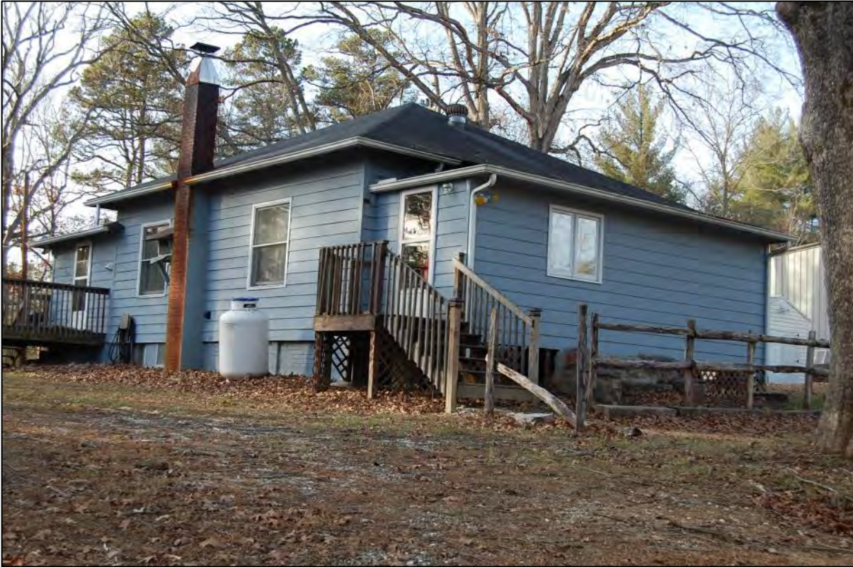
AECOM #46 - 1803 Clear Creek Rd: S side and E front (enclosed porch) elevations
