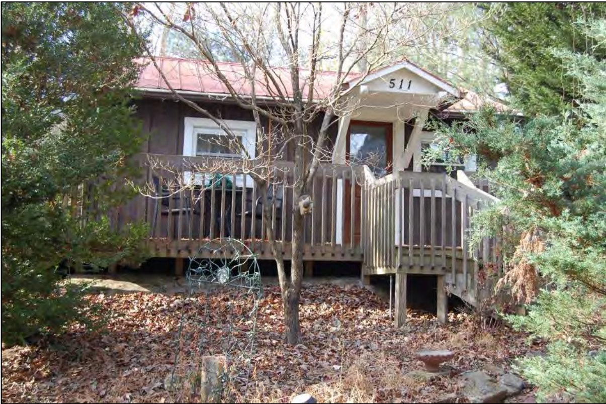
AECOM #42 - 511 Brookside Camp Rd: SE front elevation
