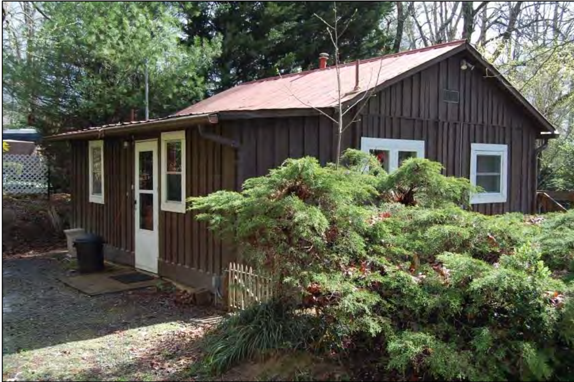
Figure 62. Northwest rear and southwest side elevations of frame cabin
