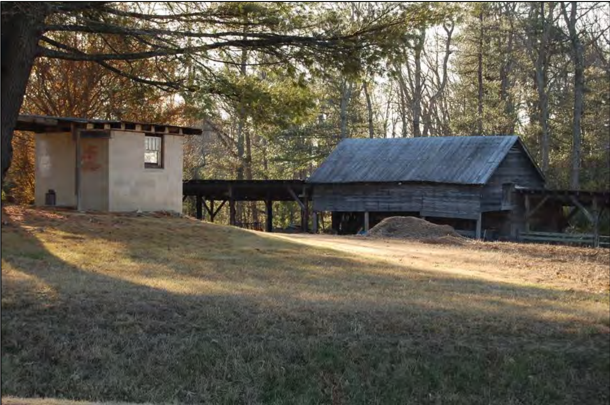
AECOM #3/HN1355 - 2886 Chimney Rock Rd: looking SW at barn and concrete-block outbuilding
