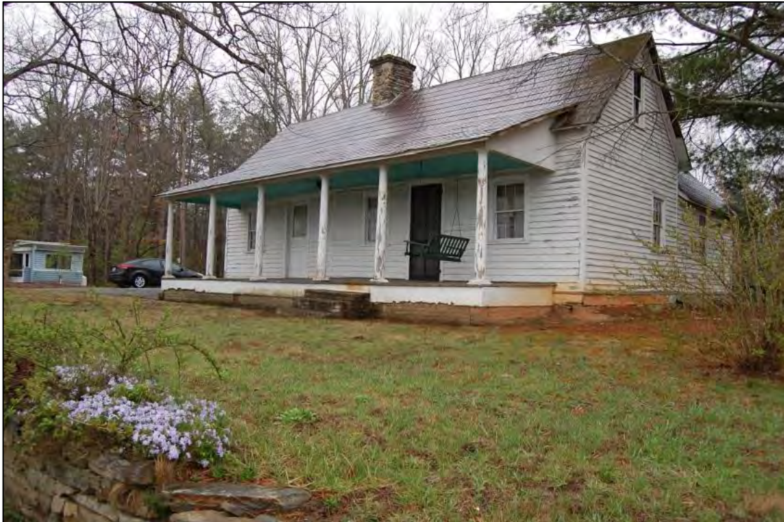
Figure 4. North front and west side elevations of house; retaining wall in foreground and mobile home at far left
