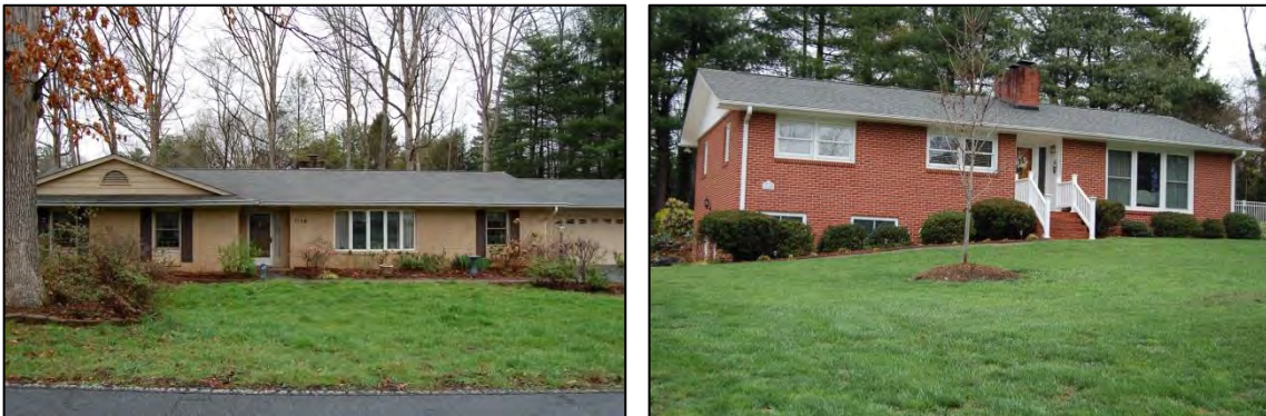
Figure 106. 3158 Florida Drive at left and 3148 Florida drive at right
