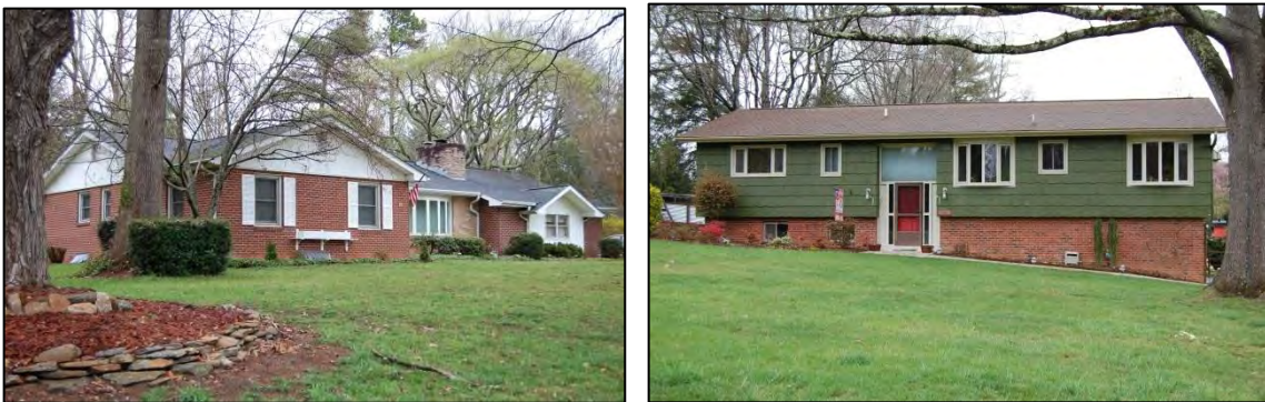
Figure 107. 3138 Florida Drive at left and 3128 Florida Drive at right
