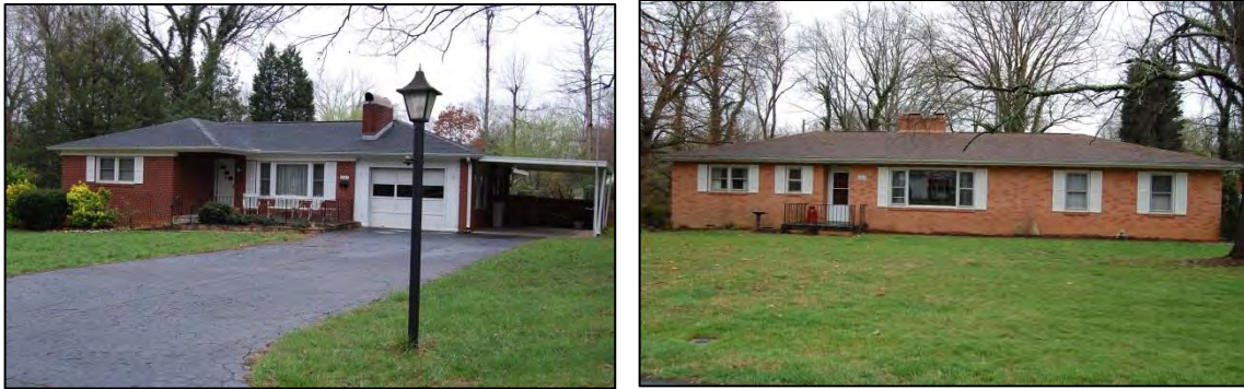
Figure 113. 3127 Florida Drive at left and 3117 Florida Drive at right
