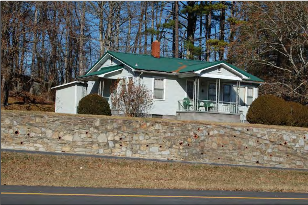
AECOM #20 - 2625 Chimney Rock Rd: SE front and SW side elevations
