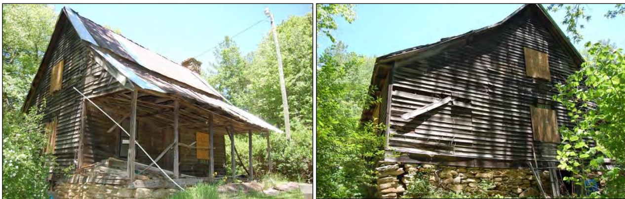
Figure 18. Riley Wall House (HN-1274): east front and south side elevations, left; south side and west rear elevations, right
