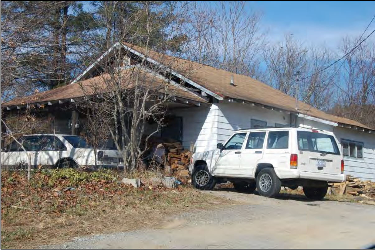
AECOM #33 - 2929 Howard Gap Rd: S front and E side elevations
