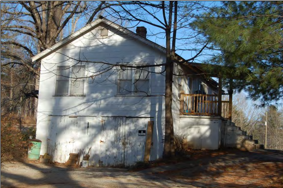
AECOM #5 - 2861 Chimney Rock Rd: S side and E front elevations
