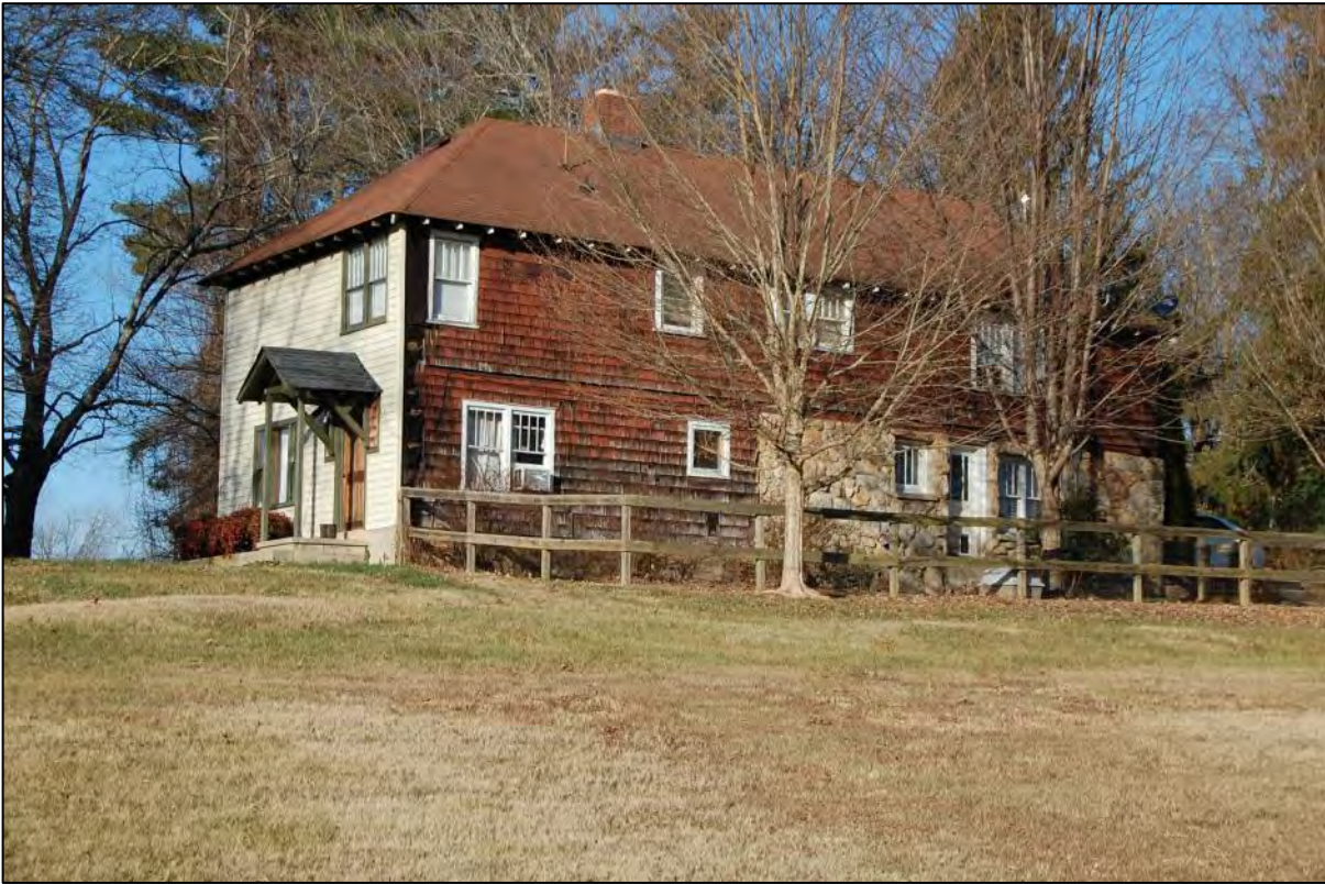
AECOM #8 - 2852 Chimney Rock Rd: S hipped and E elevations
