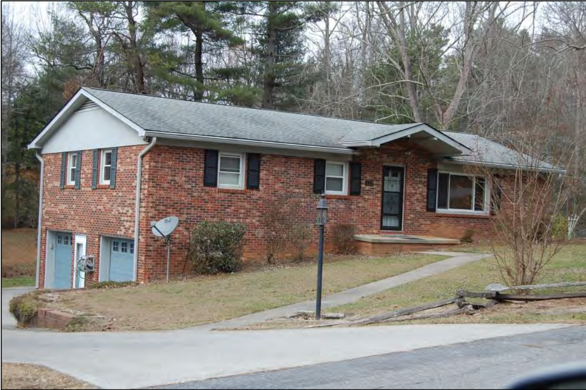
AECOM #101 - 113 Shannon Rd: E front and S side elevations
