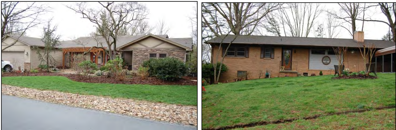
Figure 93. 3218 Florida Drive (left) and 3079 Napier Drive (right) display significant alterations to material and fenestration at their front elevations
