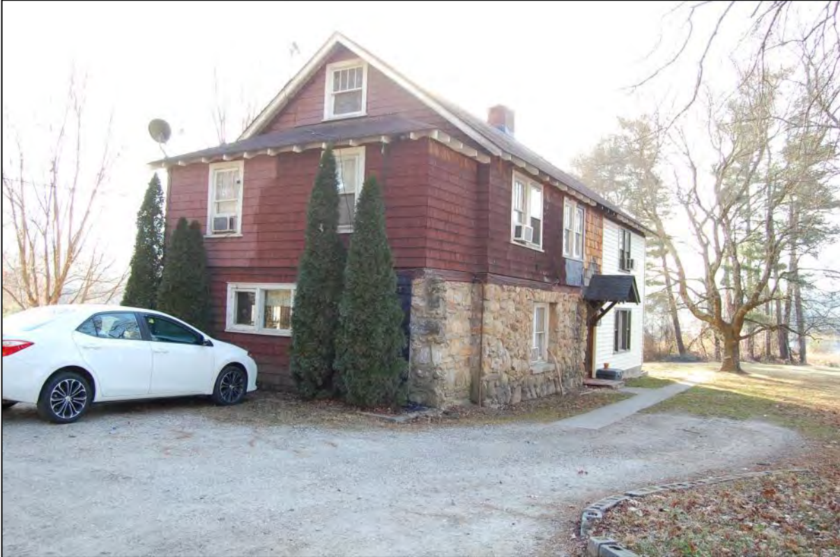
AECOM #8 - 2852 Chimney Rock Rd: N gabled and W elevations
