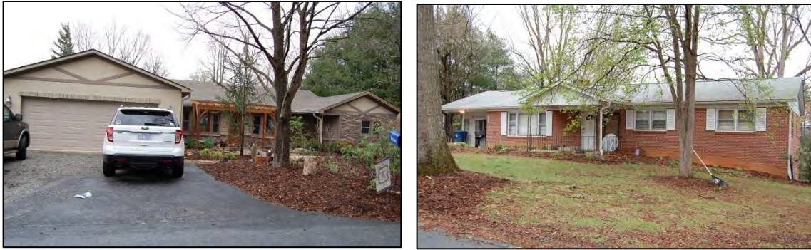
Figure 105. 3218 Florida Drive at left and 3208 Florida drive at right
