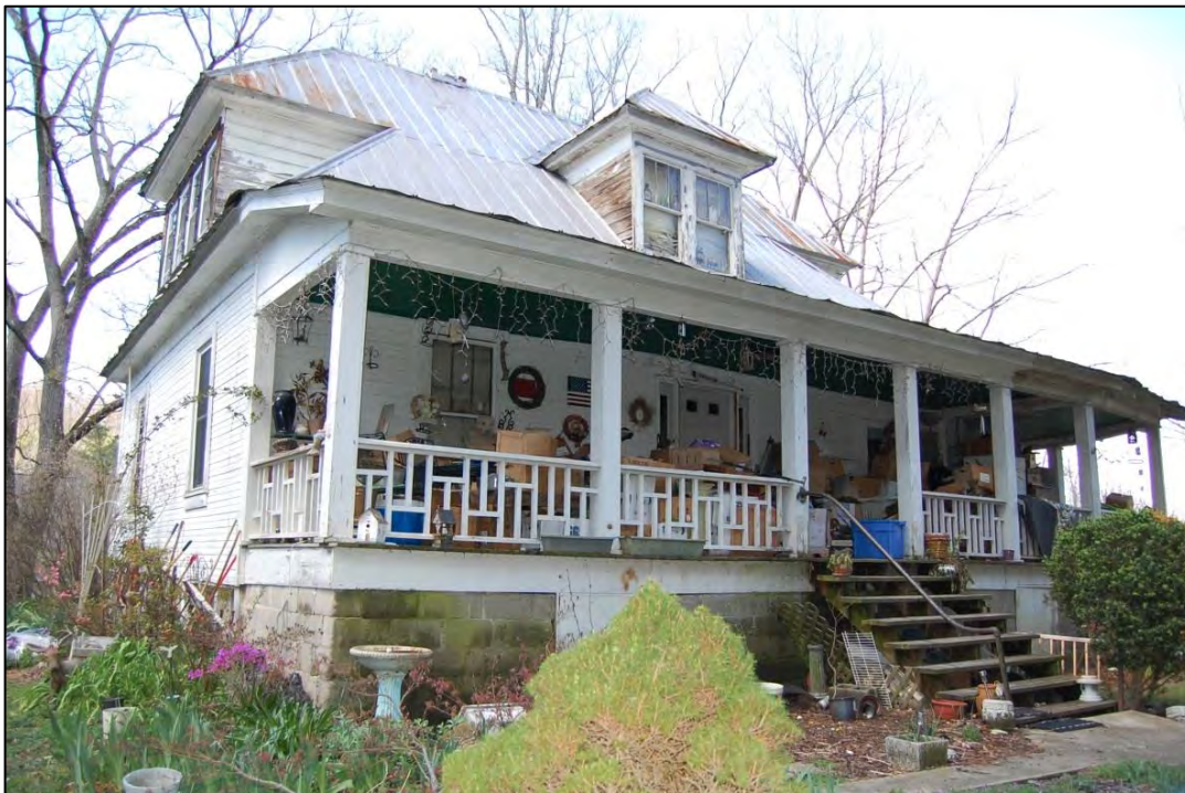
Figure 191. South side and east front elevations
