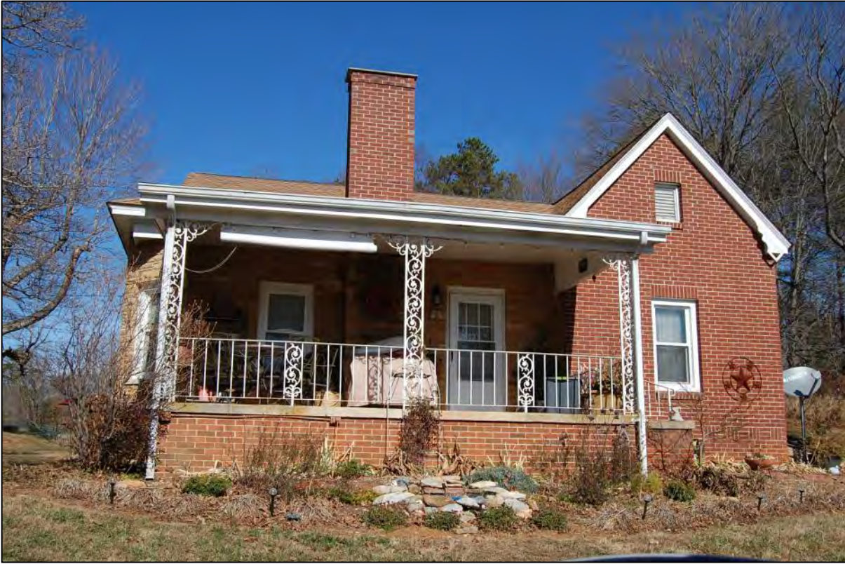
AECOM #24 - 146 Nix Rd: S front and W side elevations
