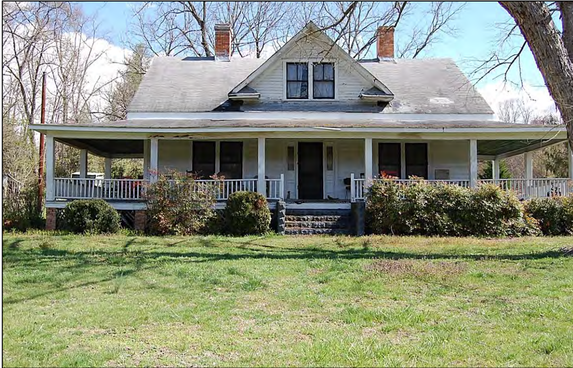
Figure 208. Southwest front elevation of house
