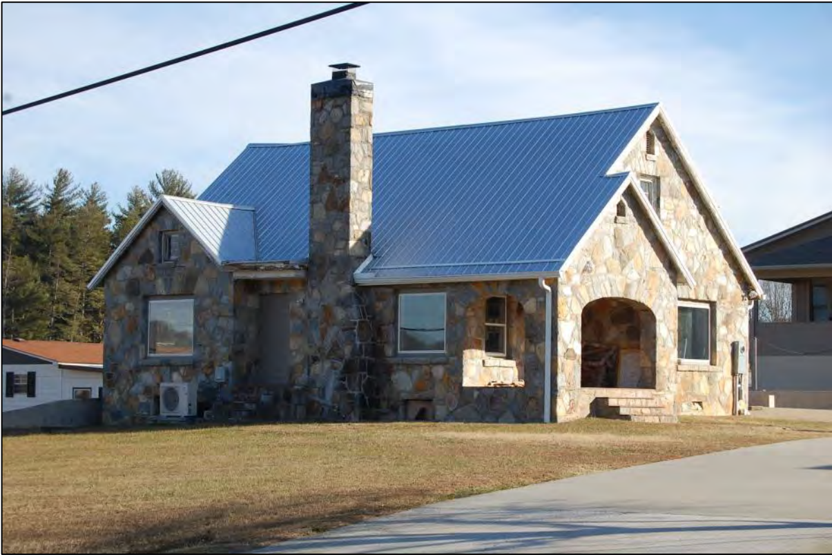
AECOM #13 – 384 Suitland Rd: gable-end S and long W elevations
