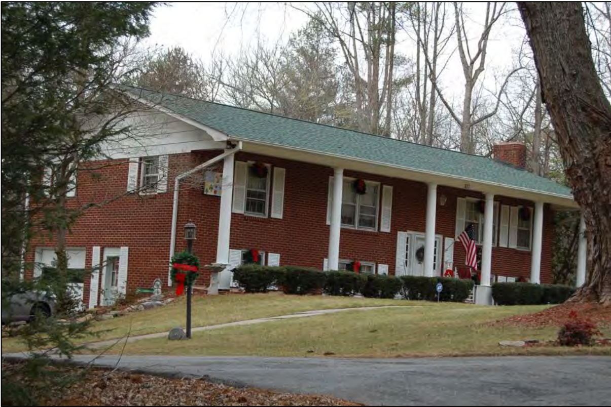
AECOM #116 - 107 Castleton Ln: E front and S side elevations
