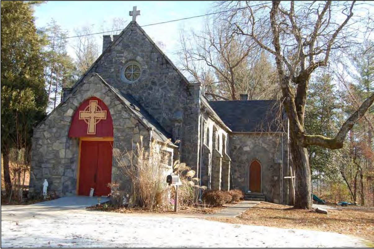
AECOM #16a - 186 St Marys Dr: W front and E side elevation of church
