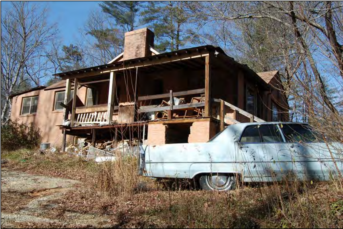
AECOM #32 -3100 Howard Gap Rd: S side and E front elevations
