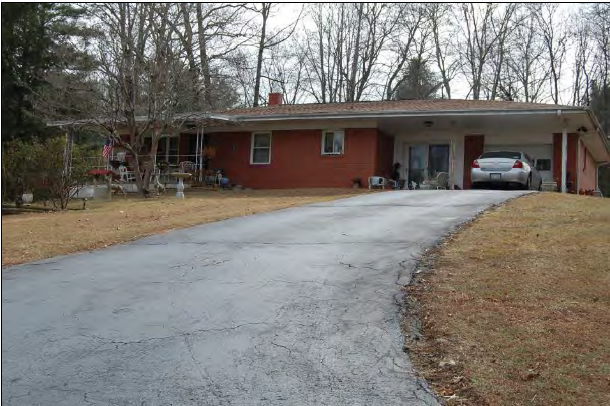
AECOM #94 - 110 May Dr: N front and E side elevations
