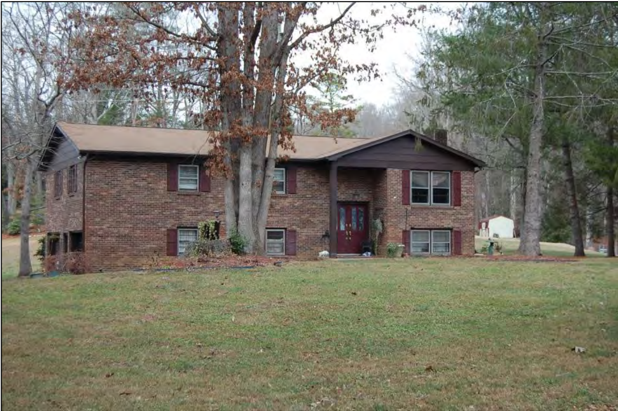
AECOM #122 - 202 Castleton Ln: S front and W side elevations
