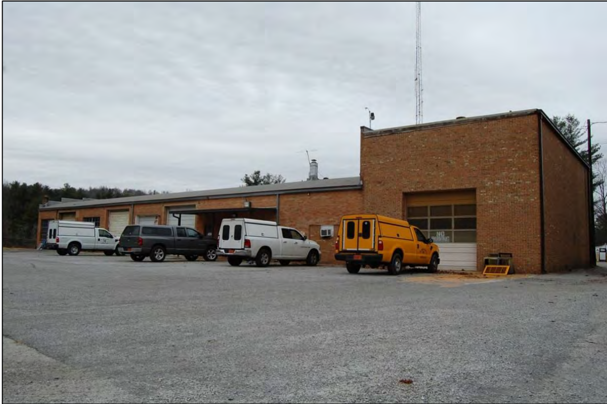
Figure 181. North and east elevations of garage; note later, taller, bay at right (north)
