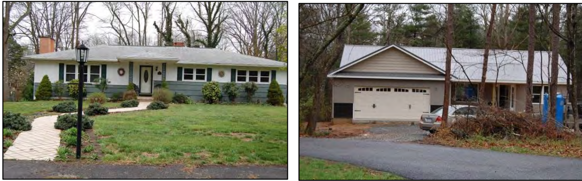
Figure 114. 3107 Florida Drive at left and 3087 Florida Drive at right
