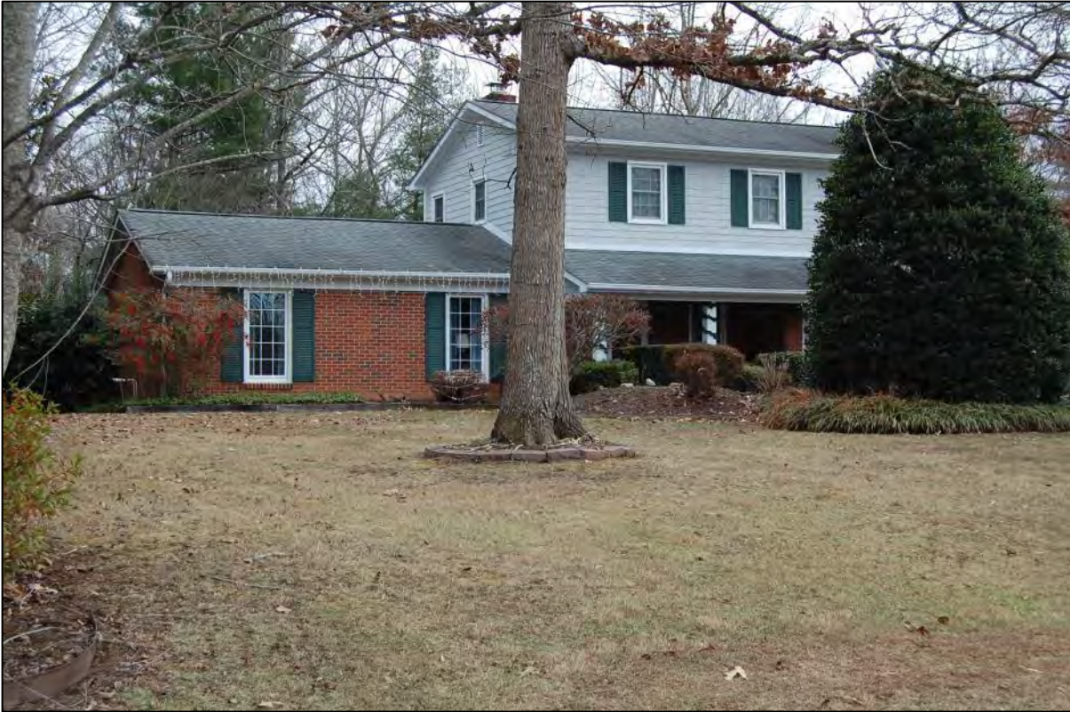
AECOM #109 - 122 Castleton Ln: W front and N side elevations
