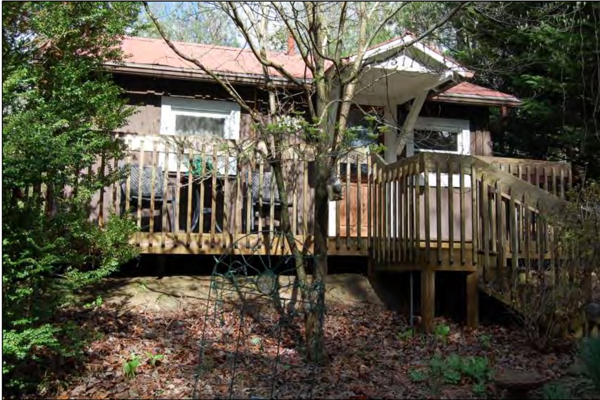
Figure 60. Southeast front elevation of frame cabin
