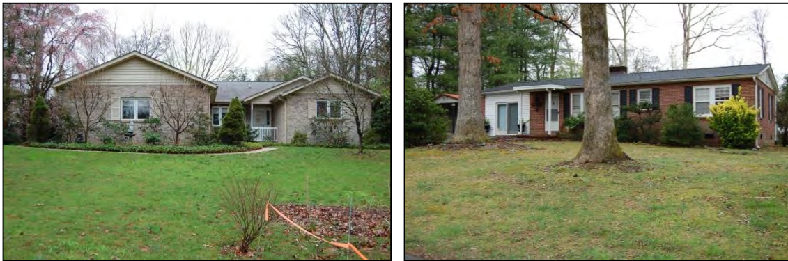
Figure 102. 3129 Cardinal Lane at left and 3119 Cardinal Lane at right
