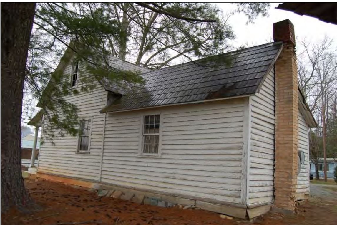
Figure 8. West side and south rear elevations of house
