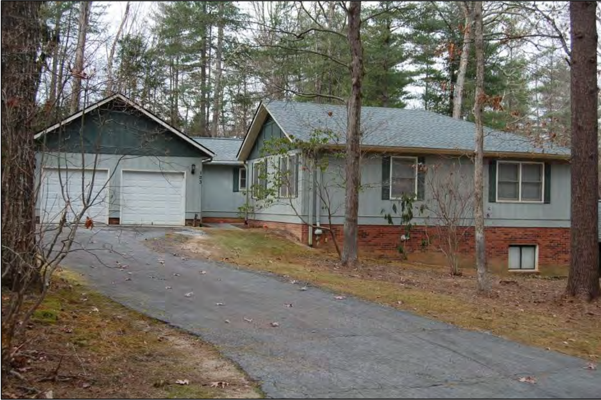
AECOM #79 - 123 Nob Hill Rd: S front (entry not visible) and E side elevations
