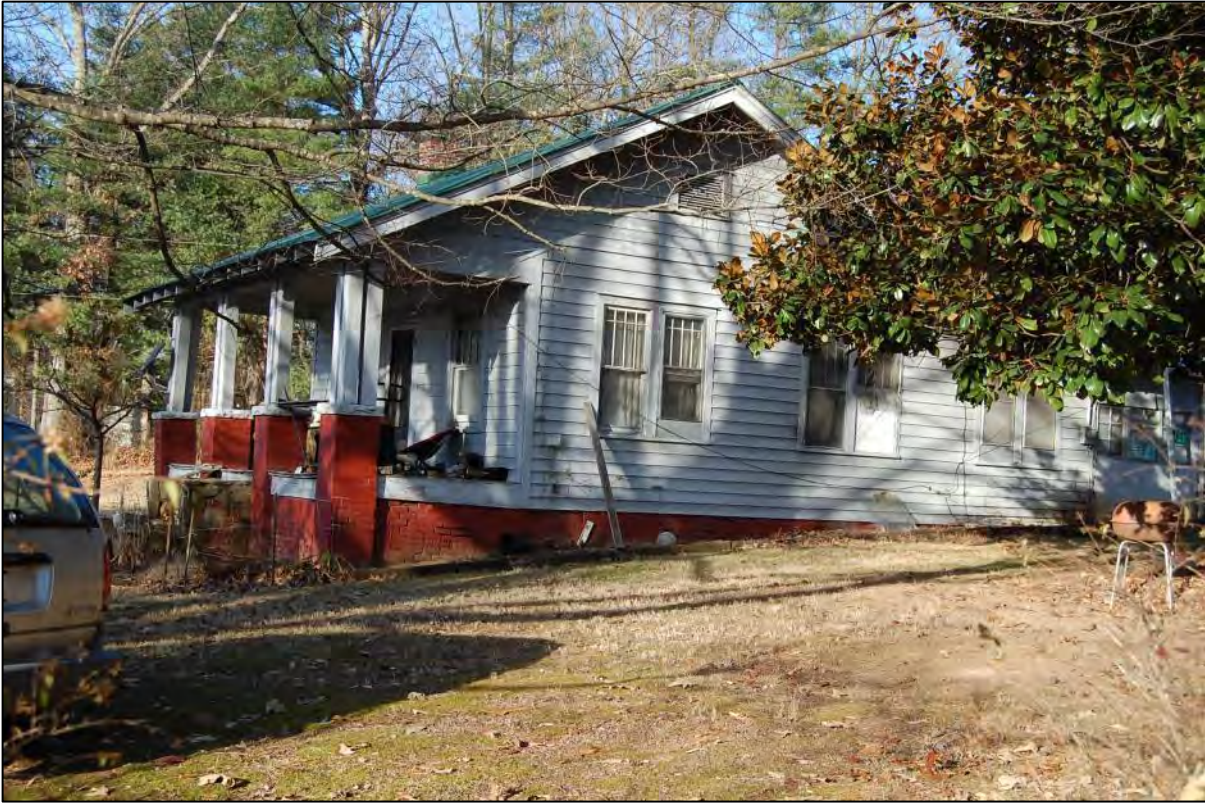
AECOM #6 - 2859 Chimney Rock Rd: E side and S front elevations
