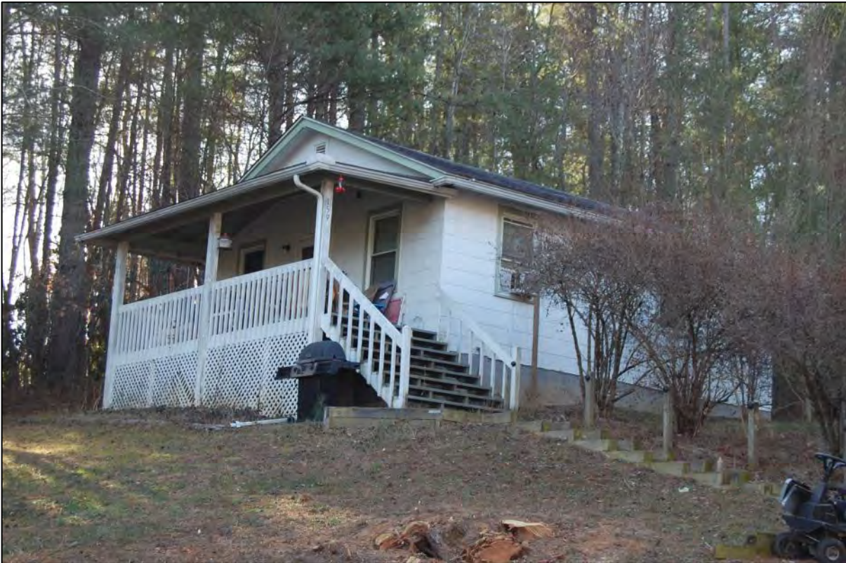
AECOM #28 - 159 Big Pine Rd: N front and W side elevations
