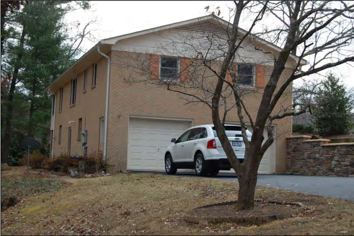
AECOM #107 - 130 Castleton Ln: N side and E rear elevations
