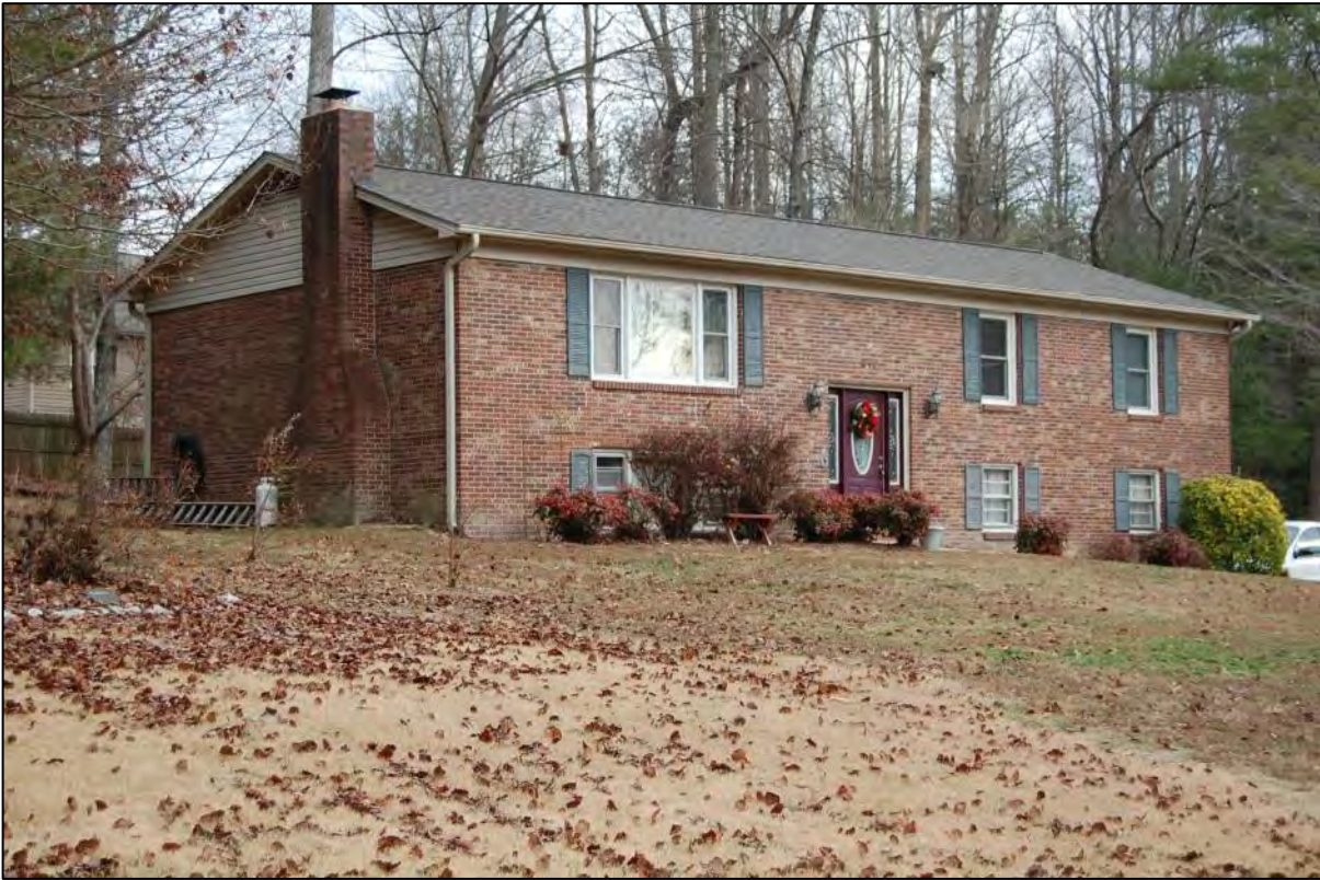
AECOM #128 - 210 Shannon Rd: W front and N side elevations
