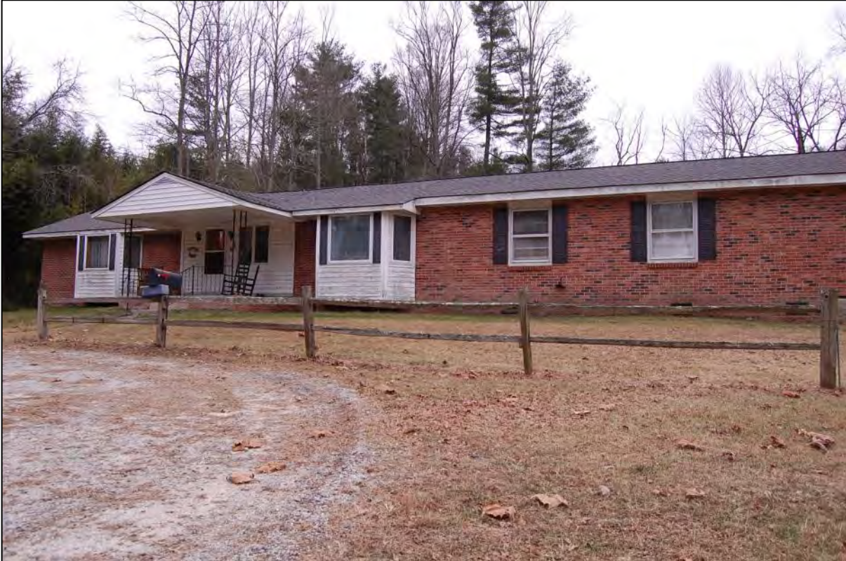
AECOM #60 - 809 Stoney Mountain Rd: N front elevation
