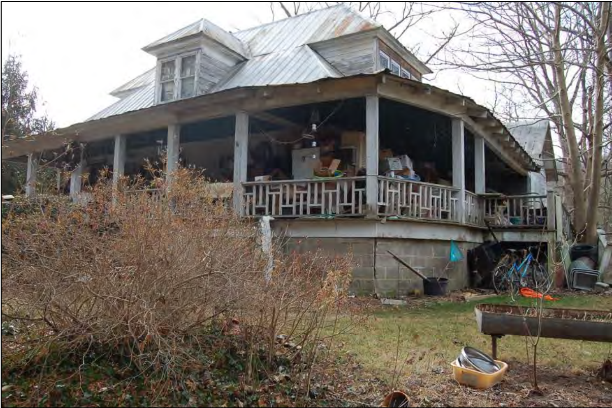
AECOM #97 - 2839 Haywood Rd: E front and N side elevations
