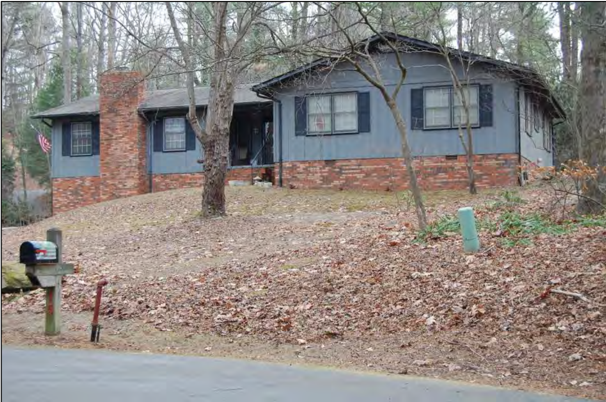
AECOM #90 - 15 Alton Way: N front and W side elevations
