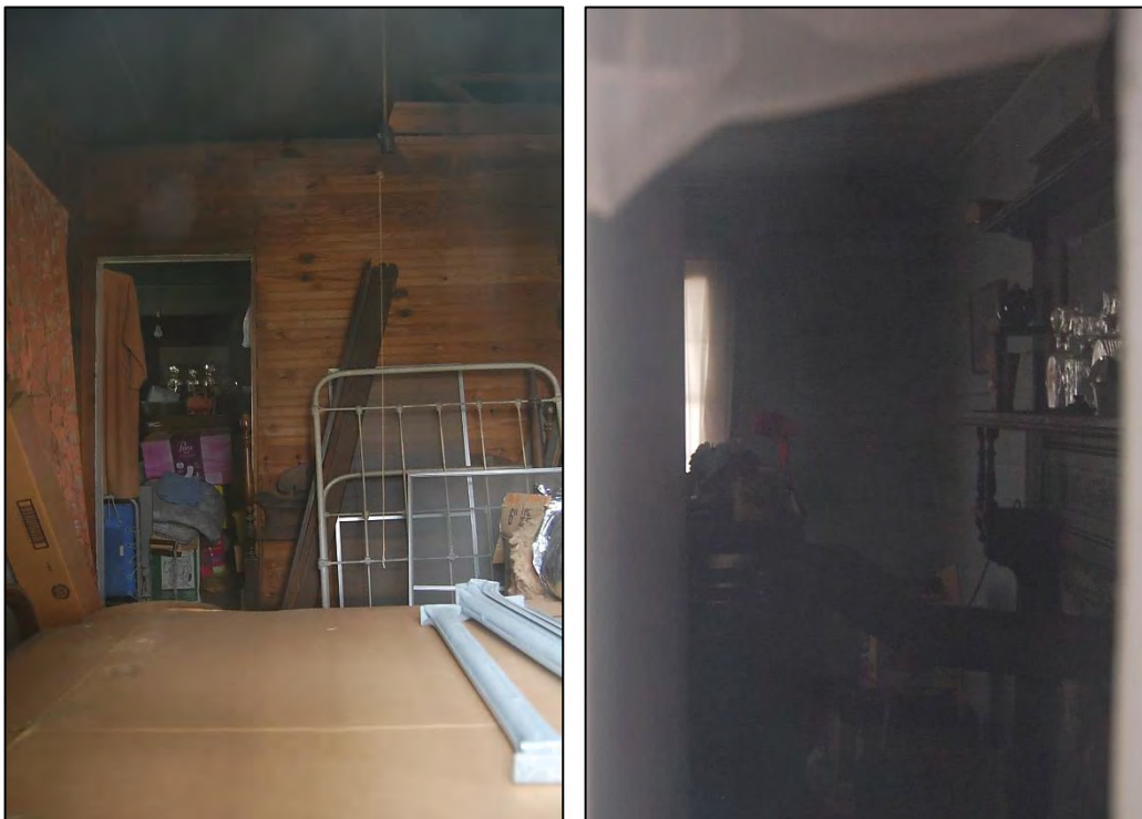
Figure 10. Bedroom or parlor and beadboard partition wall at left; flush boards and Queen Anne-style mantel in hall at right
