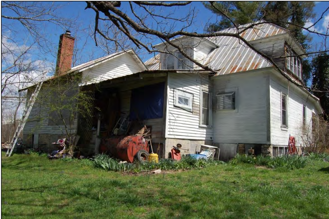
Figure 195. West rear and south side elevations
