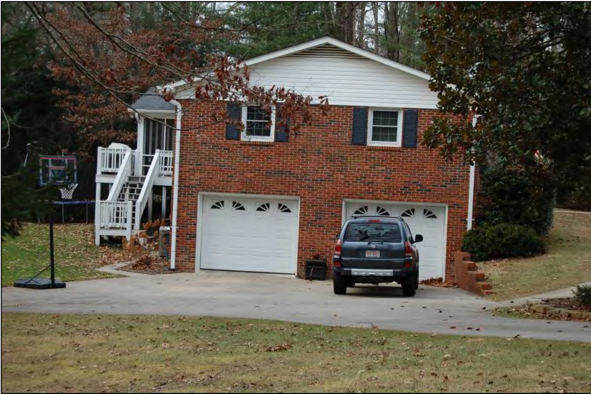
AECOM #106 - 215 Shannon Rd: E front and N side elevations
