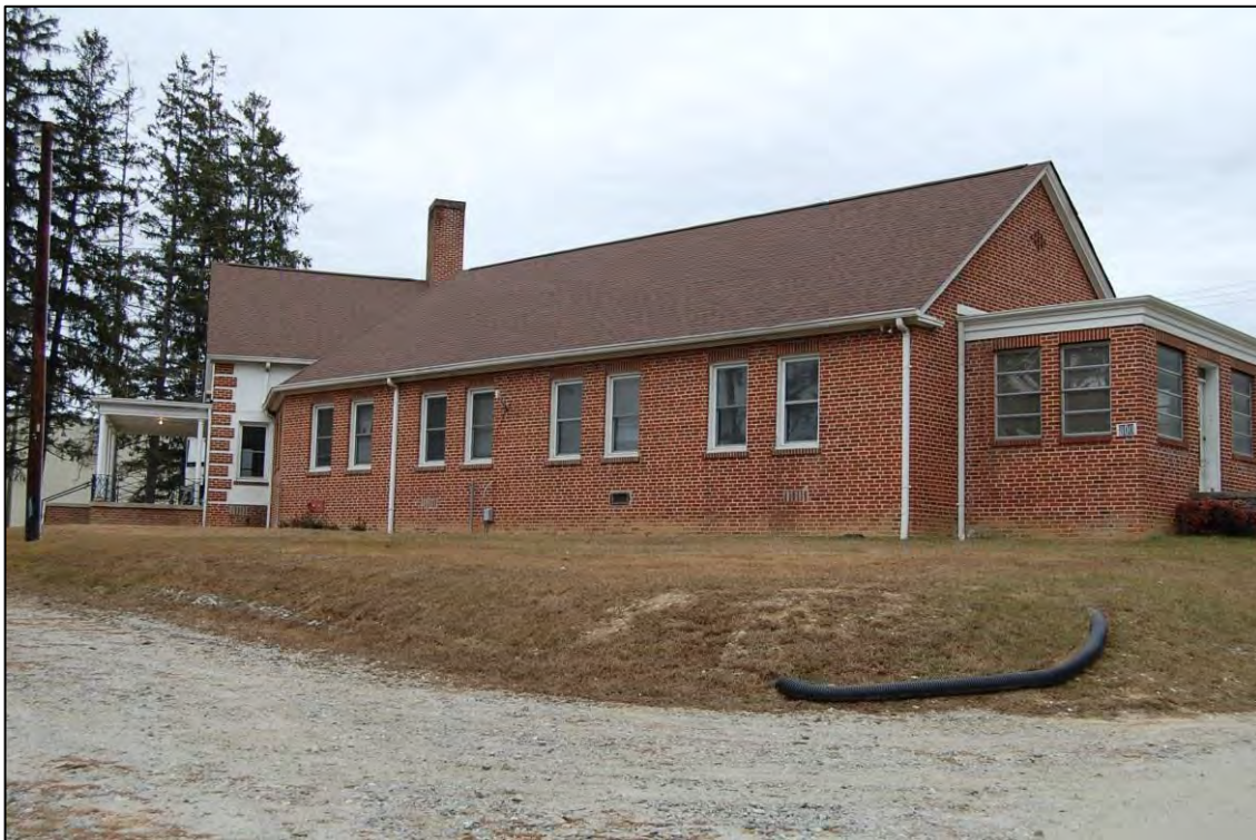
Figure 165. Looking north at former residential block’s southern wing with principal entry at left and original sunroom at right
