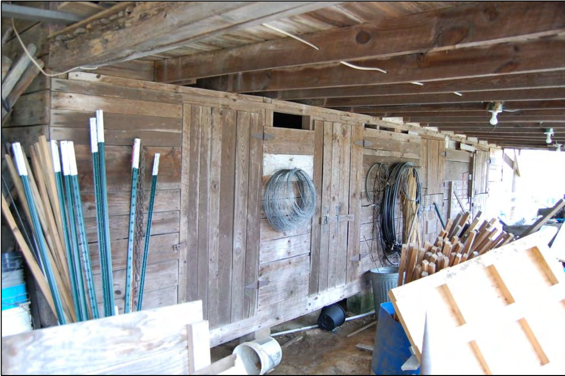
Figure 12. Looking southeast at front elevation of barn with stall doors
