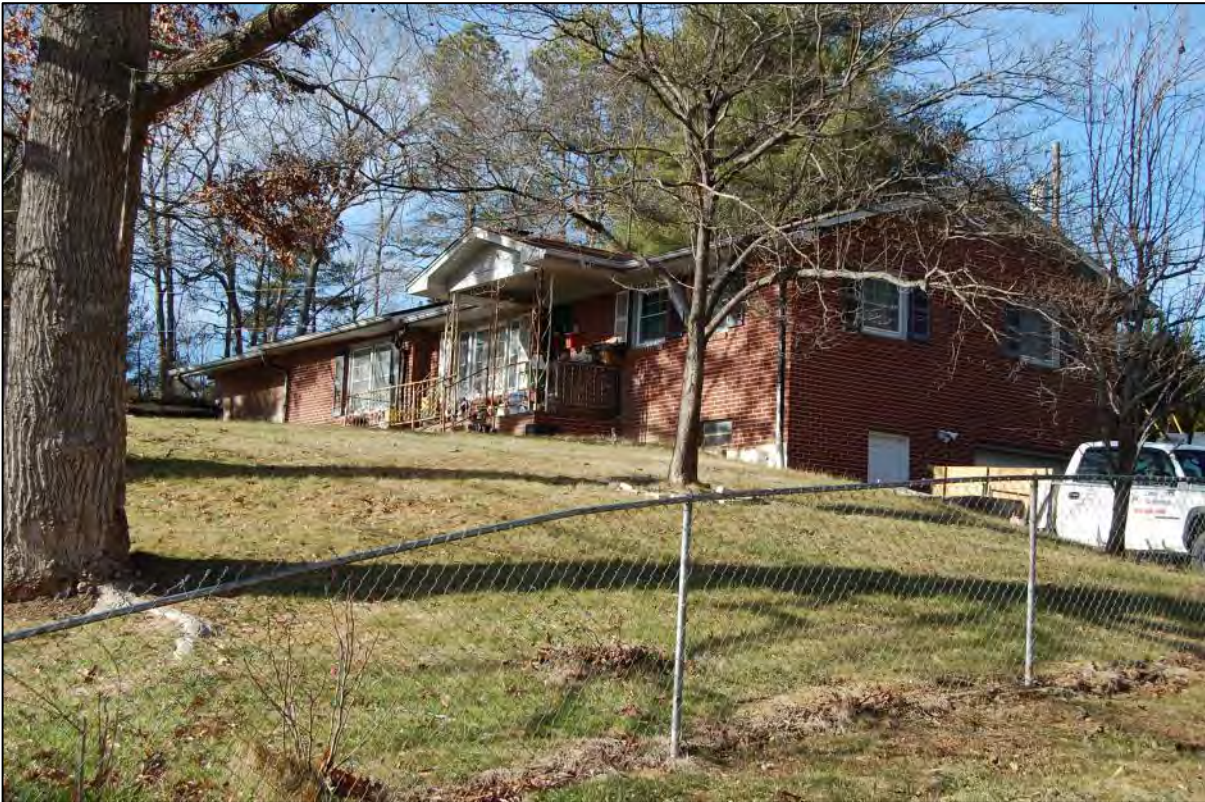
AECOM #38 - 2479 Howard Gap Rd: S front and E side elevations
