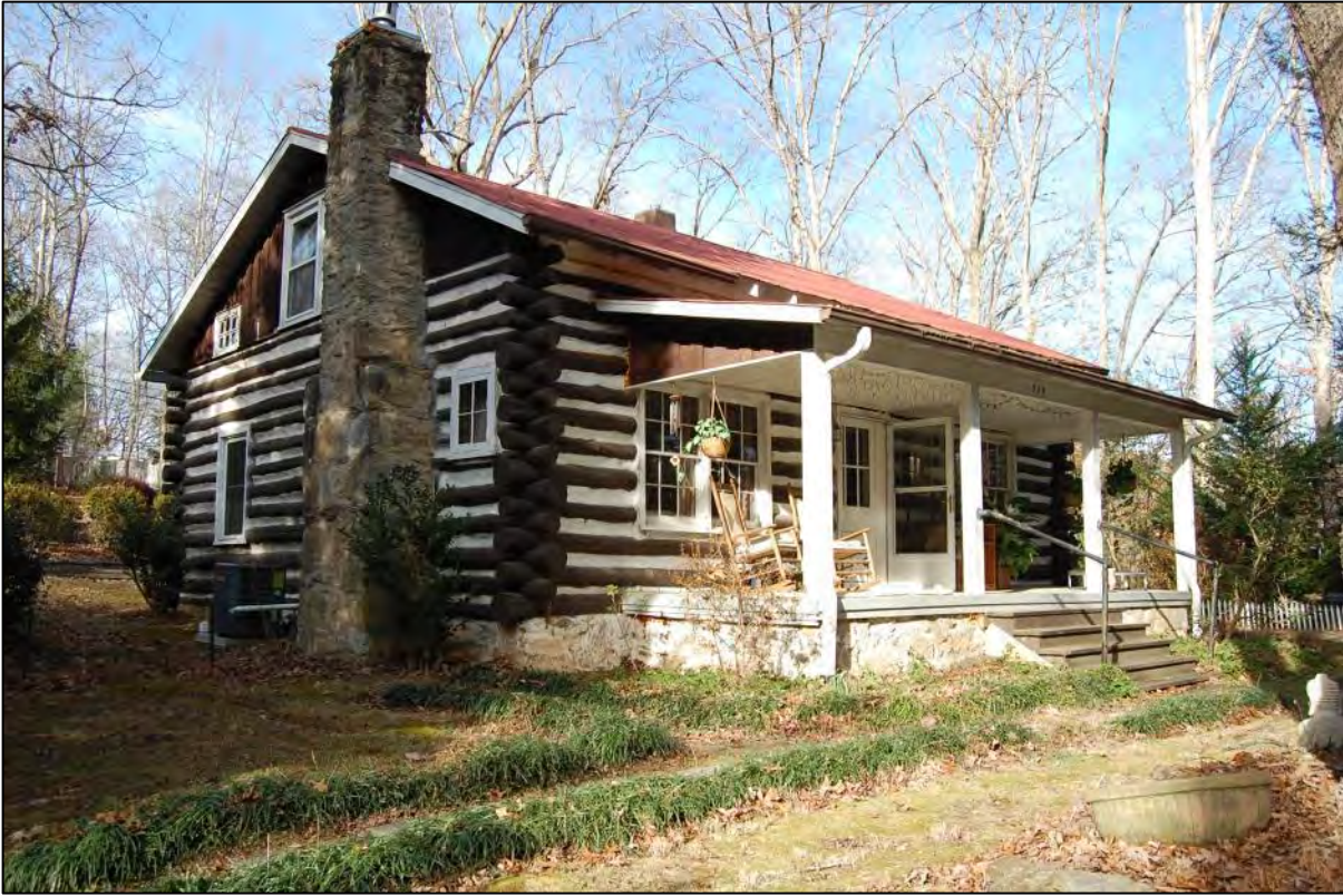
AECOM #41 - 515 Brookside Camp Rd: S front and W side elevations
