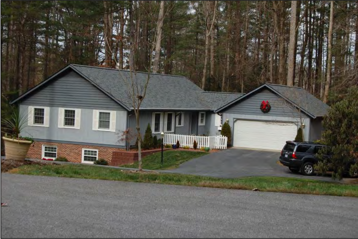
AECOM #83 - 12 Colonial Way: S front and E side elevations
