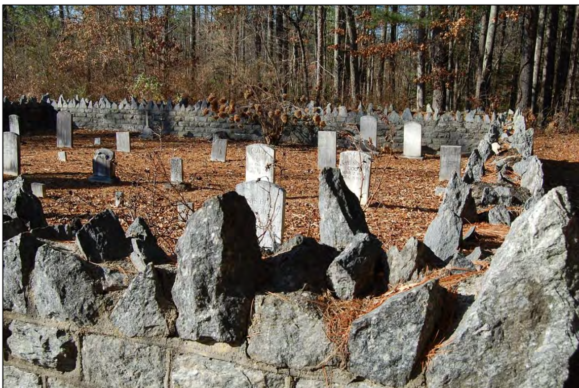
Figure 35. Looking northeast into cemetery; note width of wall topped by interior and exterior rows of pointed stones, at right
