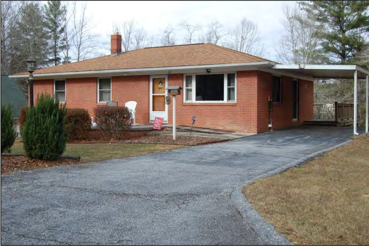
AECOM #93 - 109 May Dr: S front and E side elevations
