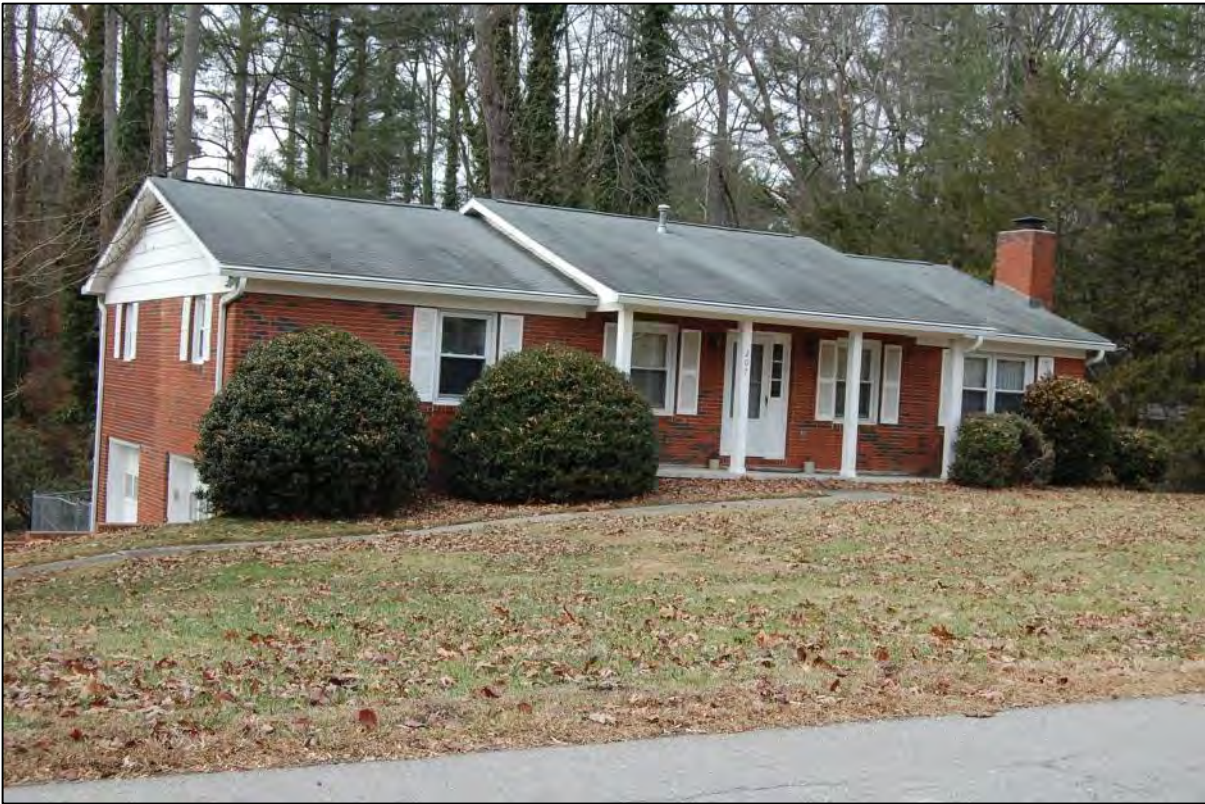
AECOM #105 - 207 Shannon Rd: E front and S side elevations
