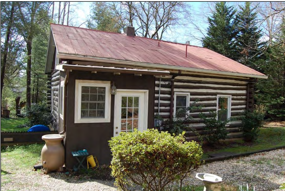
Figure 56. East side and north rear elevations of log house
