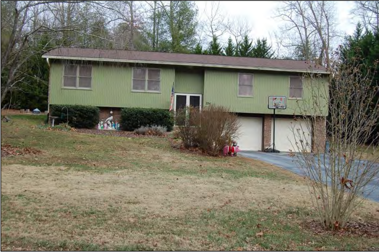
AECOM #125 - 224 Shannon Rd: W front elevation
