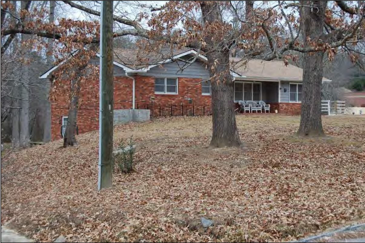
AECOM #64 – 101 Leverette Dr: S front and W side elevations
