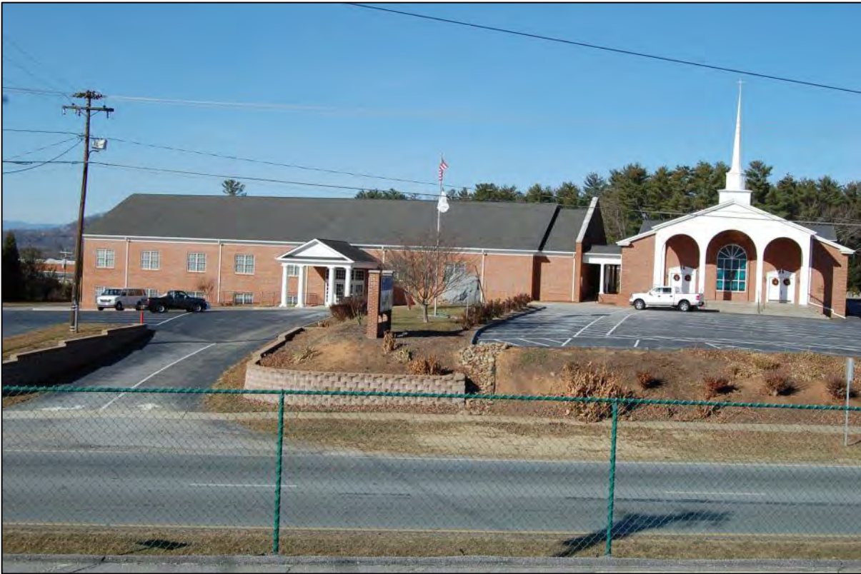
AECOM #18 - 2557 Chimney Rock Rd: E front elevation of church, at right, and education wing, at left
