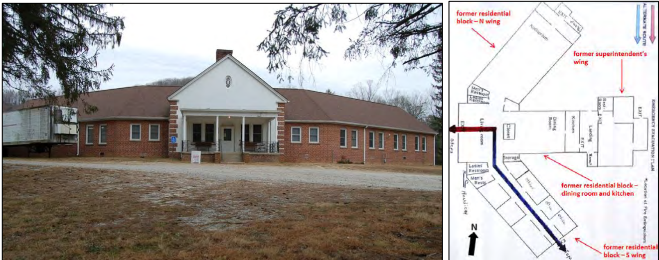
Figure 163. Looking west at front elevation of County Home’s former residential block, left; annotated plan and building footprint, right (source: County Engineering Solid Waste Division)
