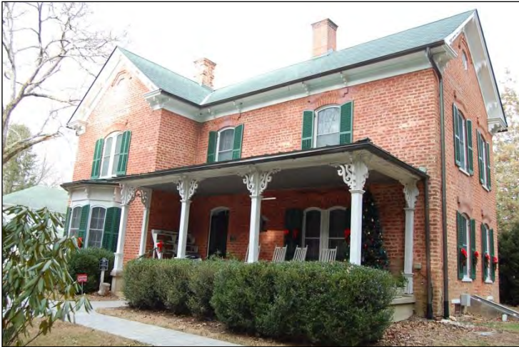
Figure 224. Southwest elevation of Moss-Johnson House
