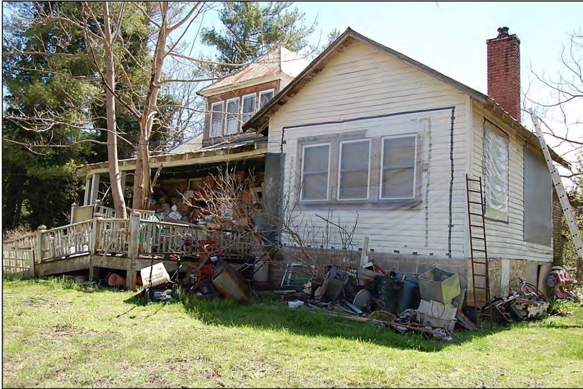
Figure 194. North side and west rear elevations
