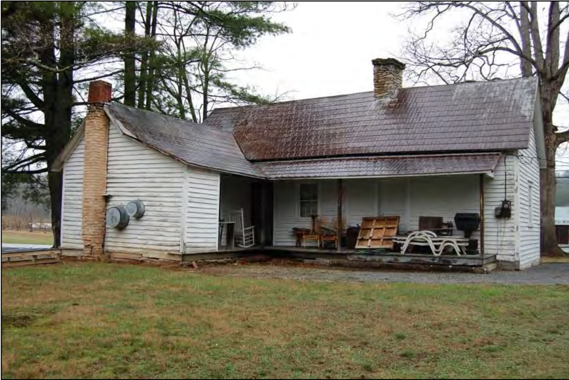
Figure 7. South rear elevation of house with ell at left
