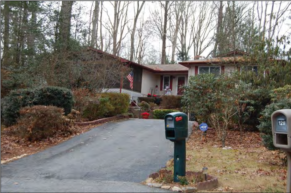
AECOM #80 - 127 Nob Hill Rd: E front elevation
