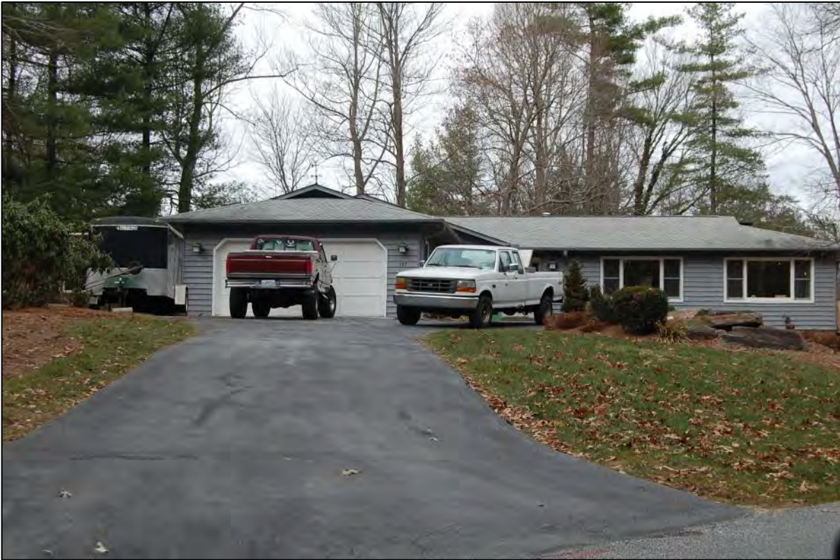
AECOM #76 - 107 Nob Hill Rd: SE front elevation
