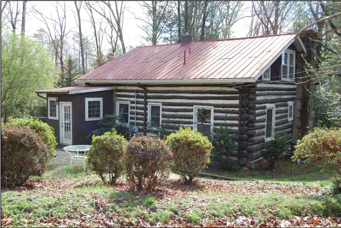
Figure 57. North rear and west side elevations of log house
