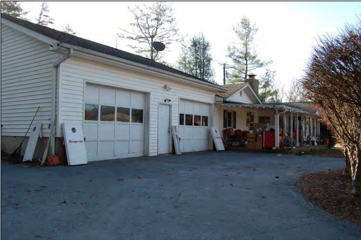
AECOM #14 - 562 Fruitland Rd: W front and N side elevations
