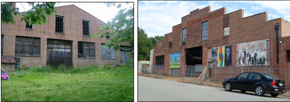
Figure 187. Carolina Coach Garage and Shop, rear elevation in 2008, at left (source: NRHP nomination), and front elevation in 2017, at right
