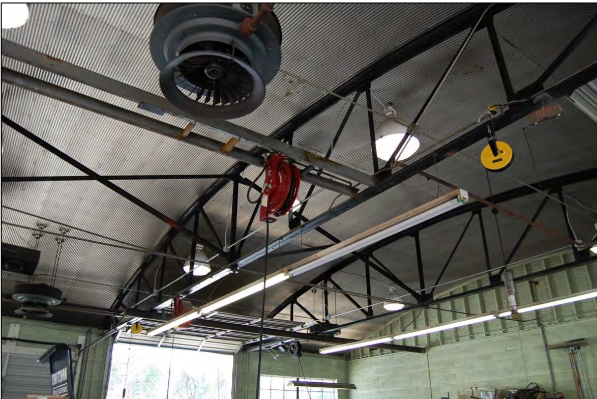
Figure 185. Garage interior, detail of trusses
