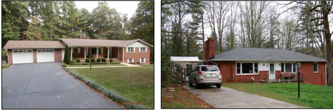
Figure 109. 3070 Florida Drive at left and 3237 Florida Drive at right
