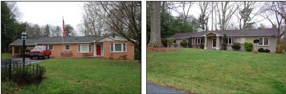
Figure 110. 3227 Florida Drive at left and 3217 Florida Drive at right
