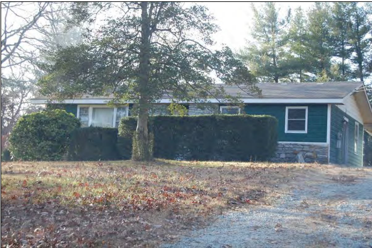
AECOM #45 (HN1932) - 1845 Clear Creek Rd: E front and N side elevations
