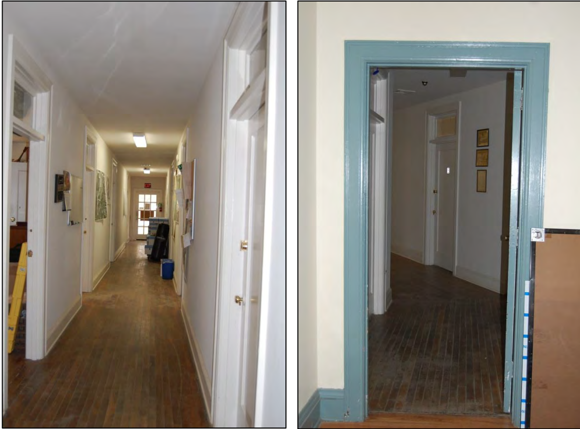
Figure 169. Corridor of former residential block south wing, at left, and view of corridor from central common room, at right
