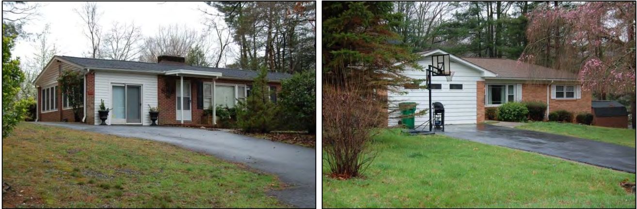
Figure 92. 3119 Cardinal Lane (left) and 3231 Magnolia Drive (right), which both feature enclosed carports, a common alteration found among houses in Grimesdale
