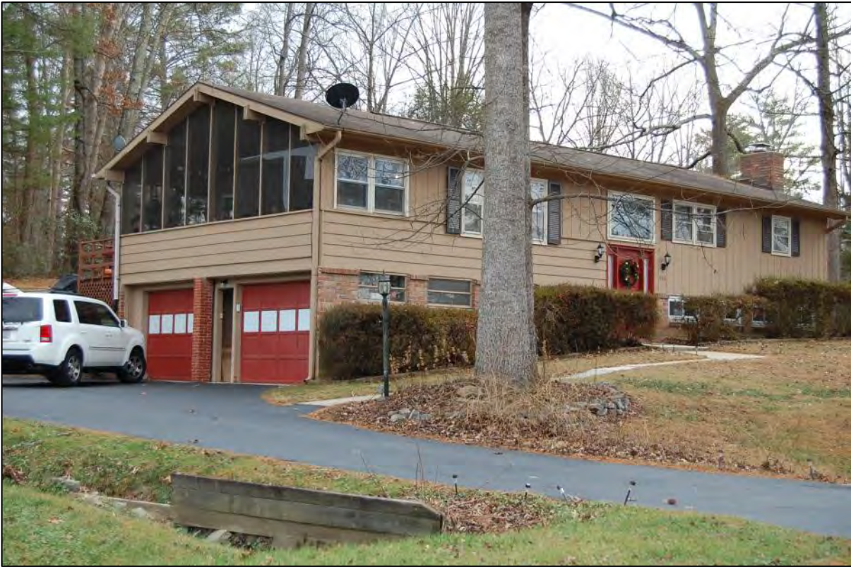
AECOM #130 - 202 Shannon Rd: W front and N side elevations
