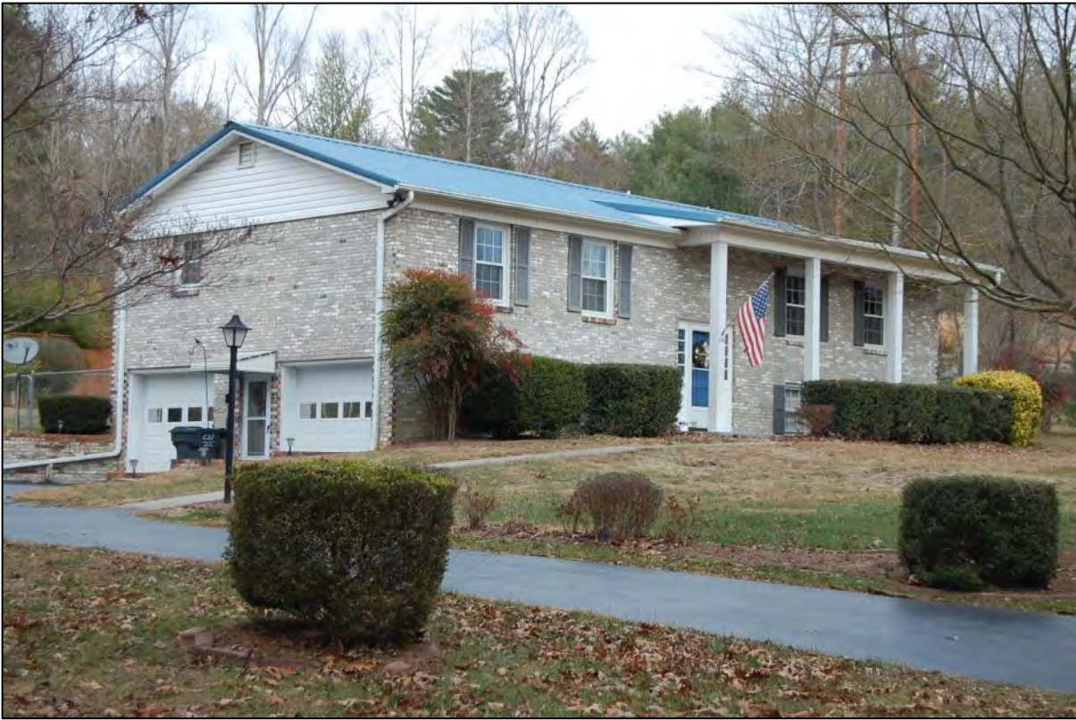
AECOM #123 - 230 Shannon Rd: S front and W side elevations
