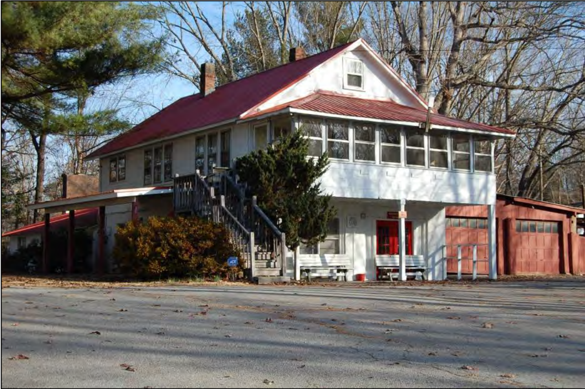
AECOM #9 - 1 Apple Orchard Rd: S front and W side of main block with later garage wing at right
