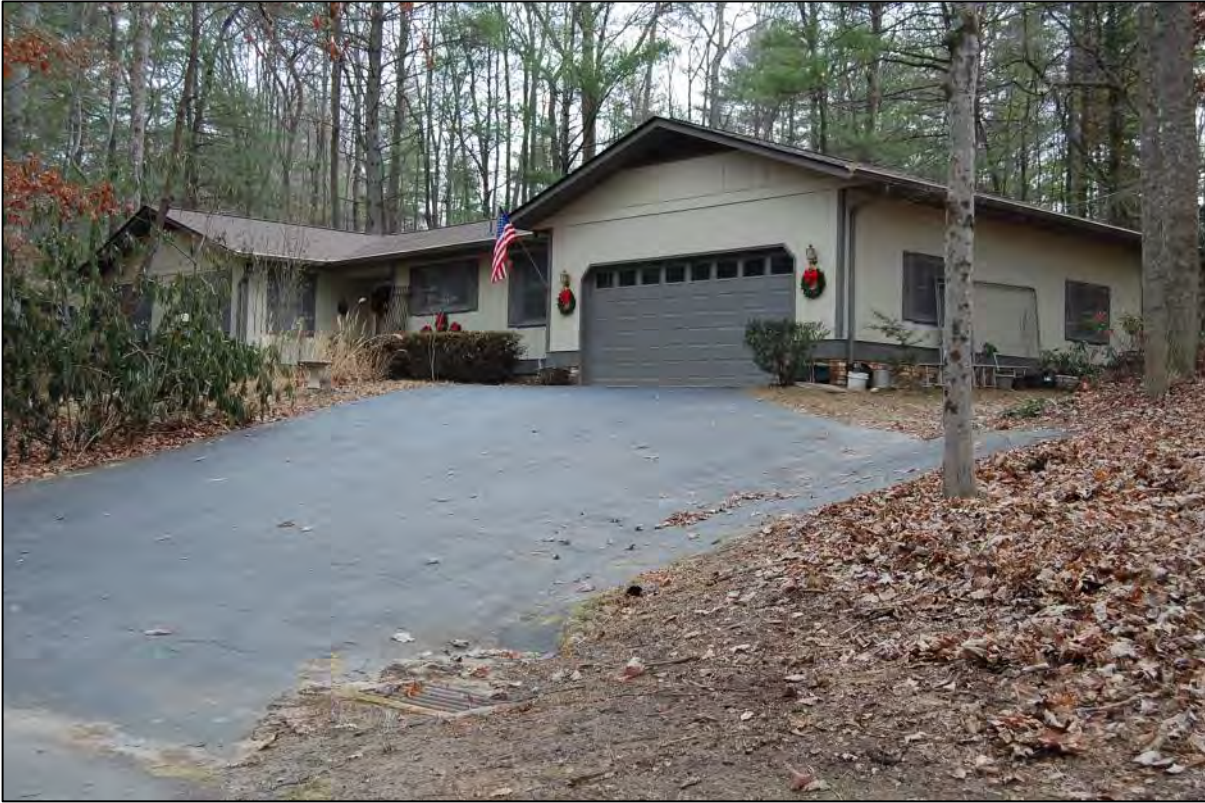
AECOM #91 - 11 Alton Way: N front and E side elevations
