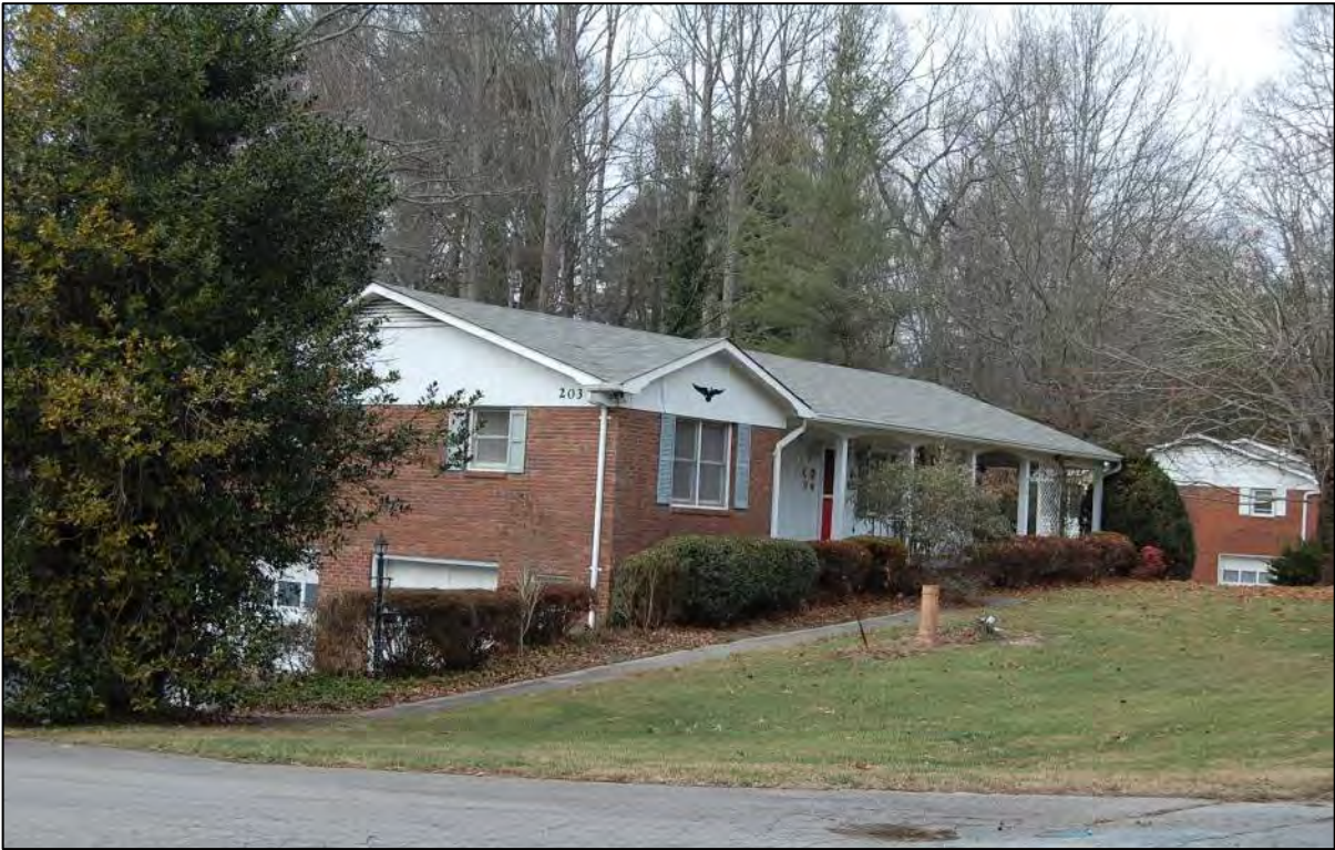
AECOM #104 - 203 Shannon Rd: E front and S side elevations
