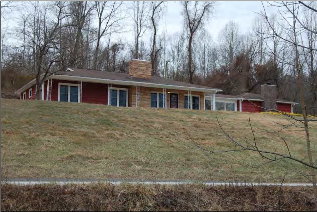
AECOM #63 – 102 Leverette Dr: N front and E side elevations
