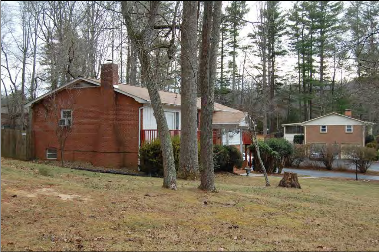
AECOM #131 - 112 Shannon Rd (at left): W front and N side elevations
