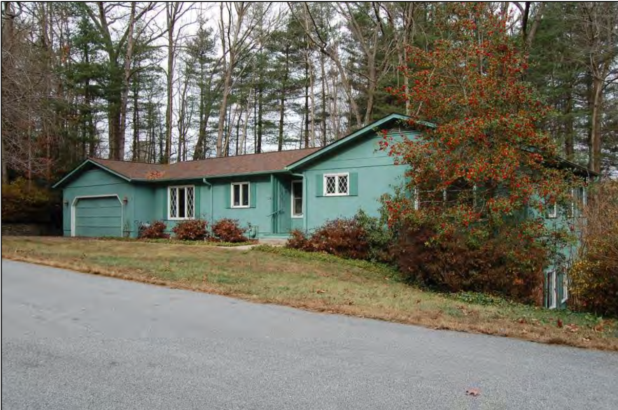
AECOM #82 - 124 Nob Hill Rd: S front and E side elevations
