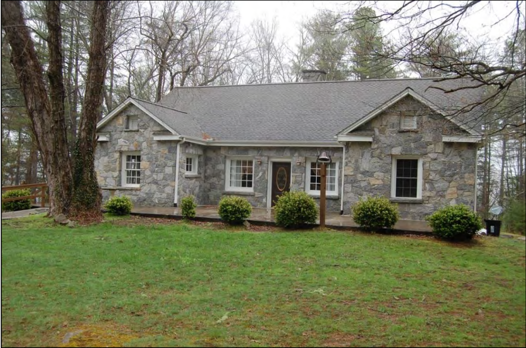
Figure 37. Southwest front elevation of house
