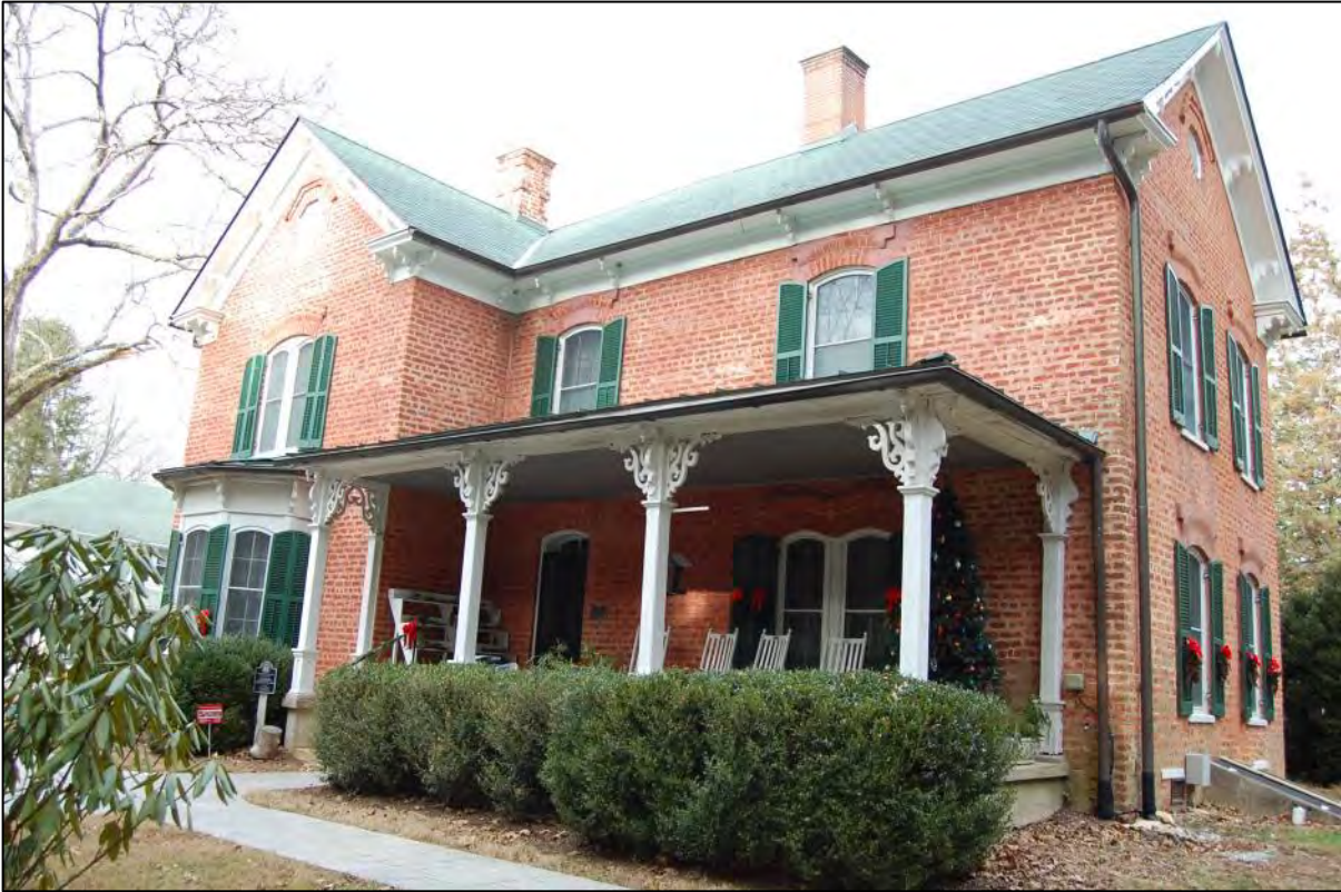
AECOM #135 (HN0043) - 3346 Haywood Rd: Moss-Johnson Farm main house SW front and SE side elevations
