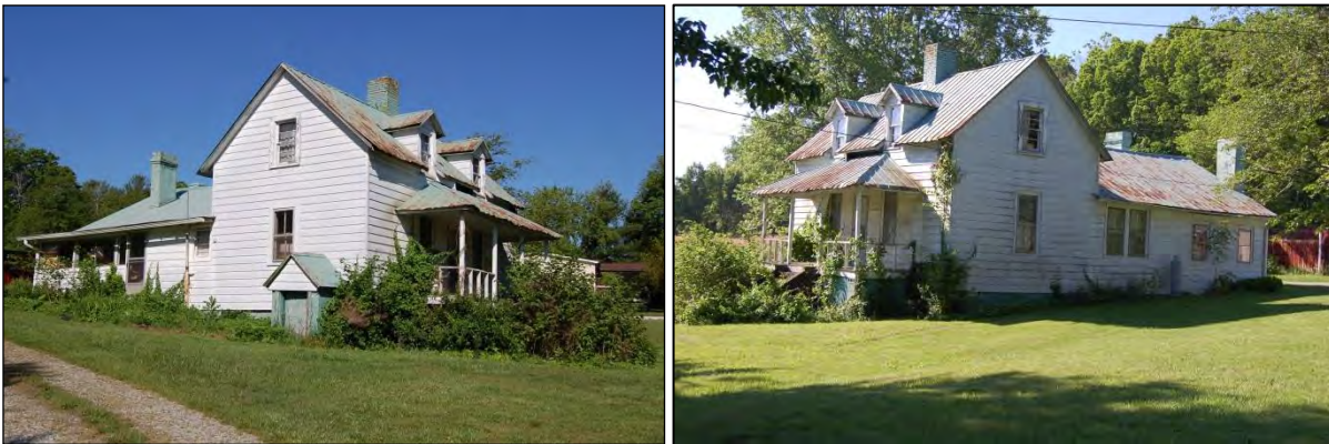
Figure 22. Frady House (HN-1146): east side and north front elevation, left; north front and west side elevation, right
