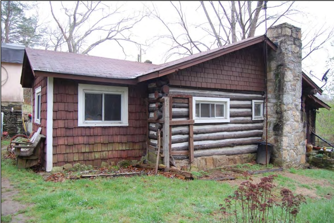
Figure 79. North side elevation of house with ell extending to east rear; gambrel-roofed shed on tall stone foundation at far left
