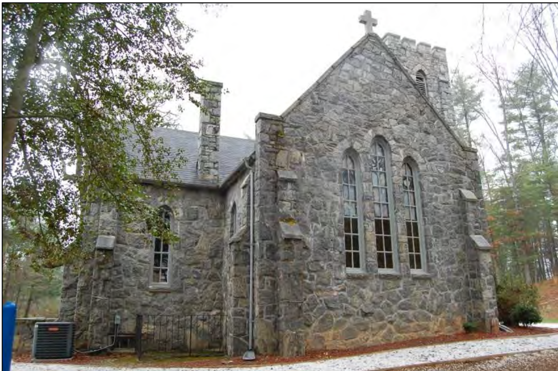
Figure 29. East rear elevation of St. Mary's Chapel
